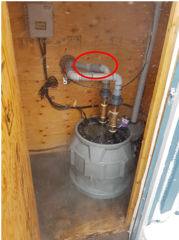
Figure 3: Wing 10 outflow to equalizer tank disconnected.
