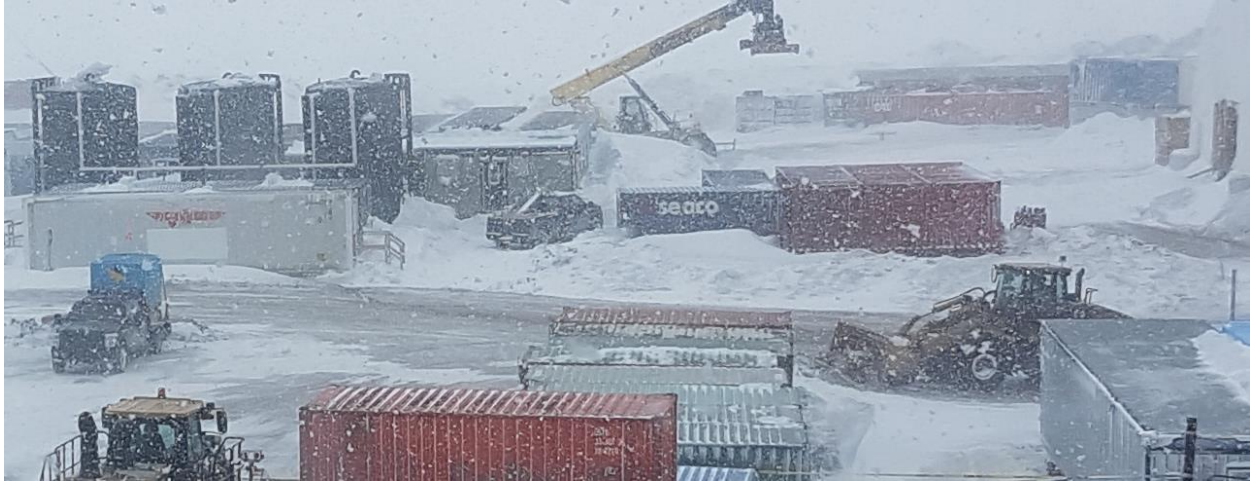
Figure 4: A loader was used to remove contaminated gravel for transport to Landfarm A.
