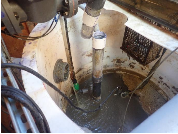
Figure 2: The pipe, which is connected to the pump inside the lift station, separated at a connection point.
