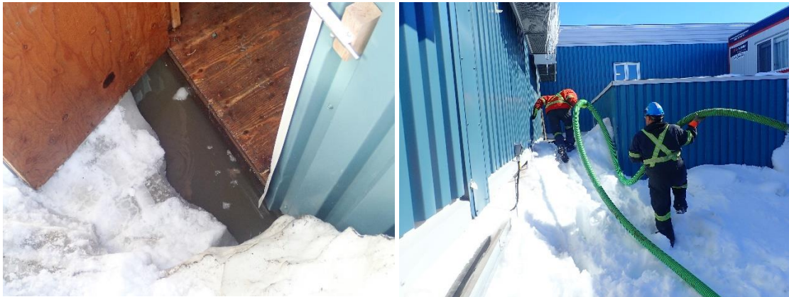
Figure 3: Standing water outside of the lift station was removed using the sucker truck.
