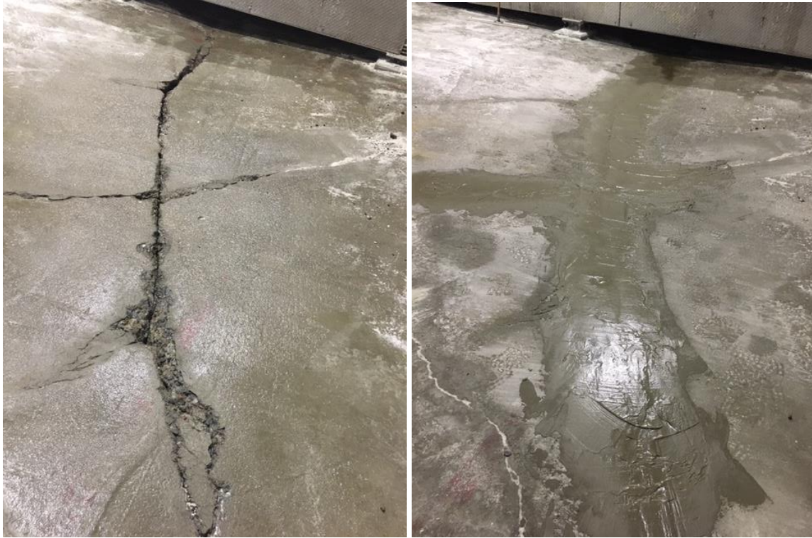
Figure 2: Cracked concrete foundation saline water flowed through (left) and repairs made 1 st March 2020 (right).
