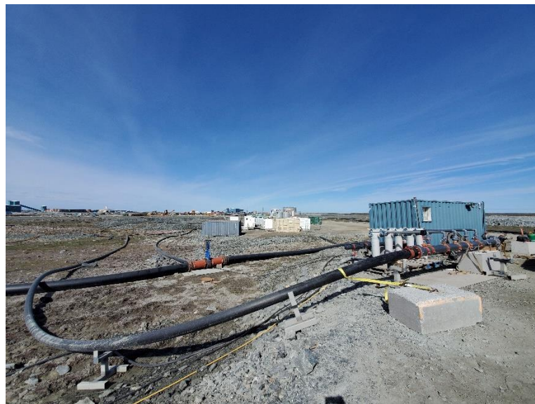
Figure 3: Piping replaced from SP3 to loading station.
