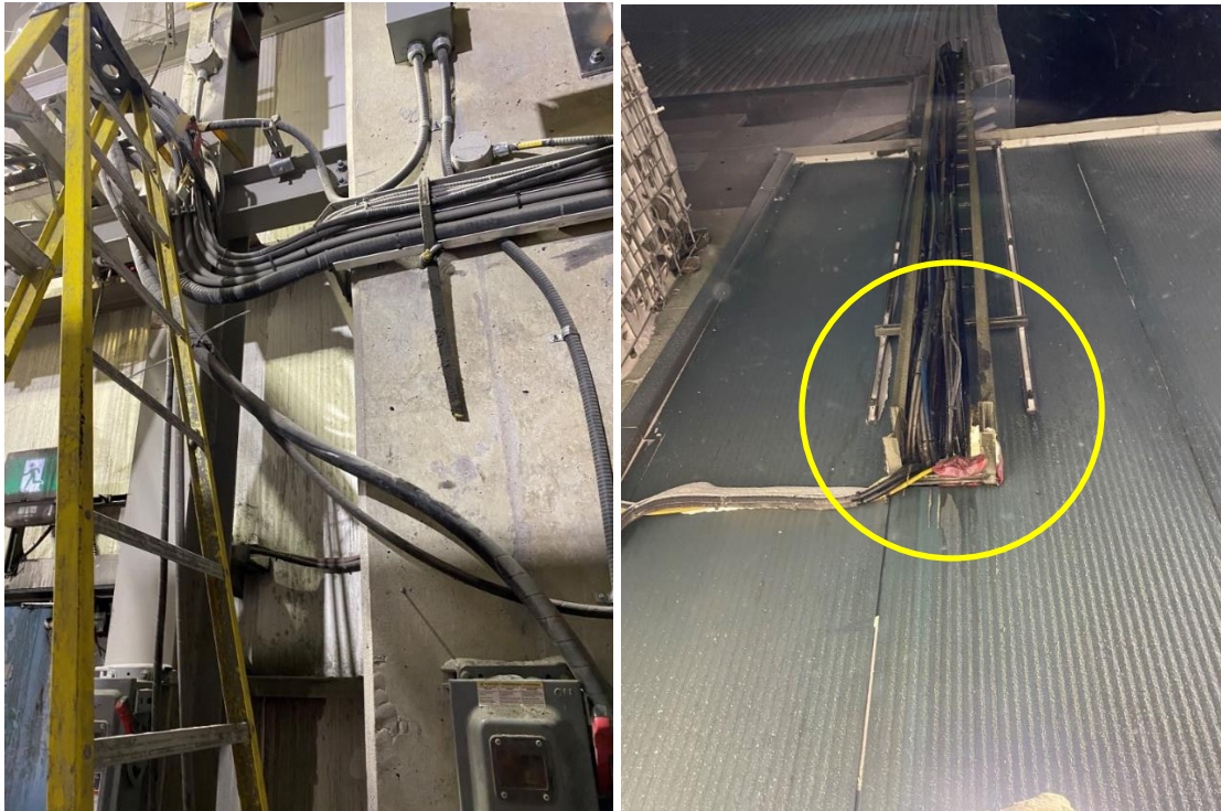
Figure 2: A hydraulic line breakage occurred on the exterior of the building (circled area).
