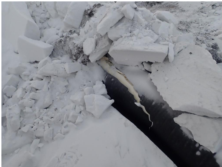
Figure 3: Damage to heat recovery waterline.
