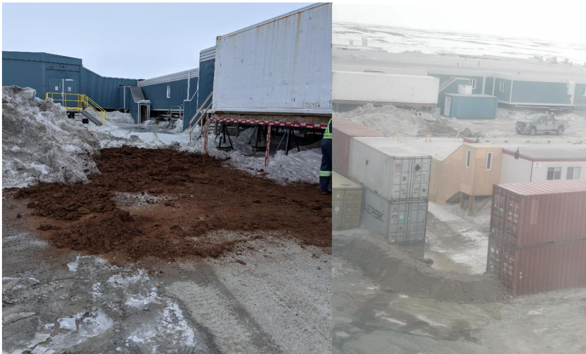
Figure 6: Clean peat/soil was used to absorb pooling water, and a temporary berm construction to mitigate downstream flow.
