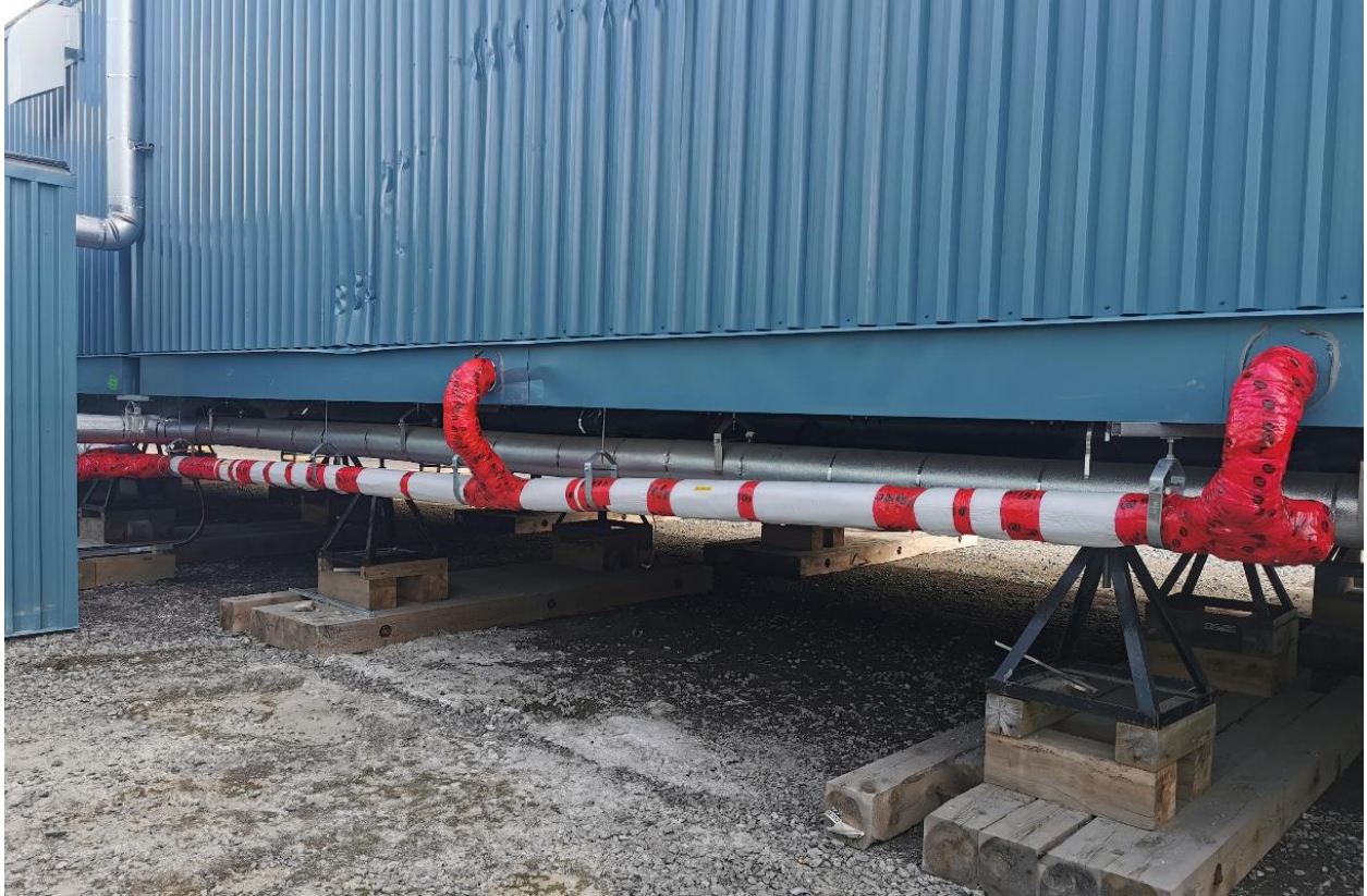
Figure 4: Clean up of the area and reinstallation of the drainpipe with heat trace and insulation.
