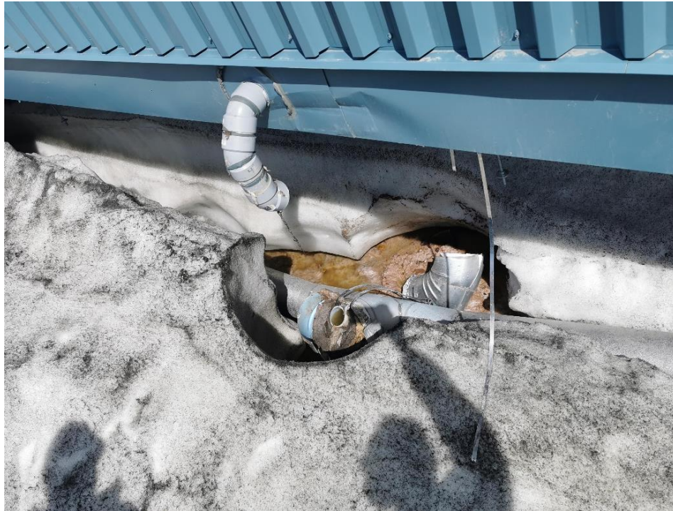
Figure 2: Drainpipe on the exterior of Wing 12 that separated from the building due to the weight of snow.
