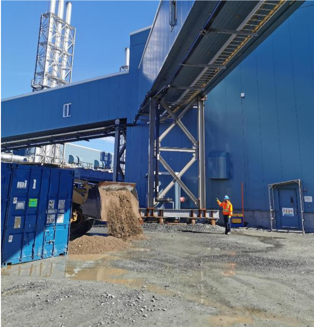
Figure 2: Sand berm being created at the south end of the spill location to contain the heat recovery water.
