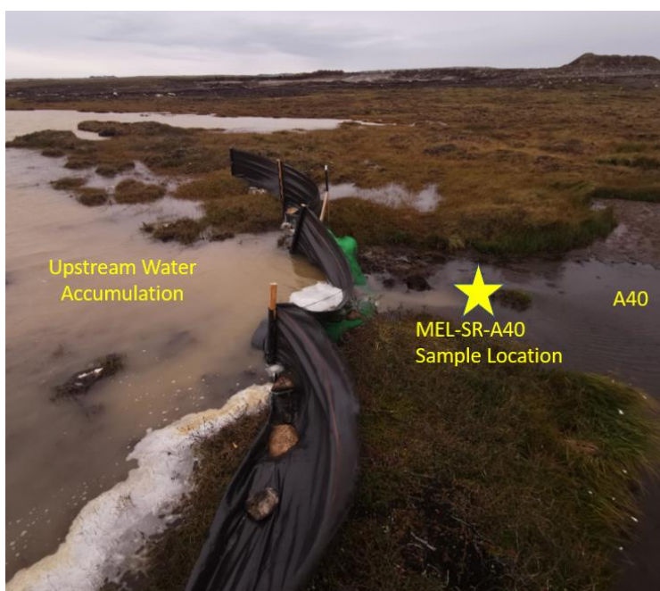
Figure 2: Installation of sediment control fence and logs. Sample location established immediately downstream of the sediment control fence.
