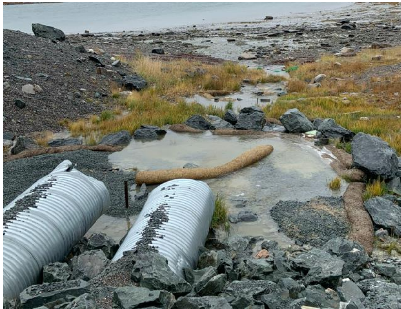
Figure 2: Sediment control at discharge
