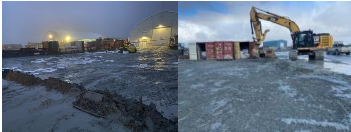
Figure 3: Containment berm and excavator clean up.
