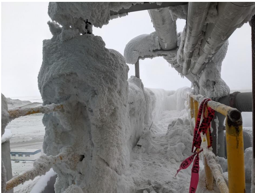
Figure 3: Pre-clean up of the overhead ice on the thickener tank (caused by humidity)
