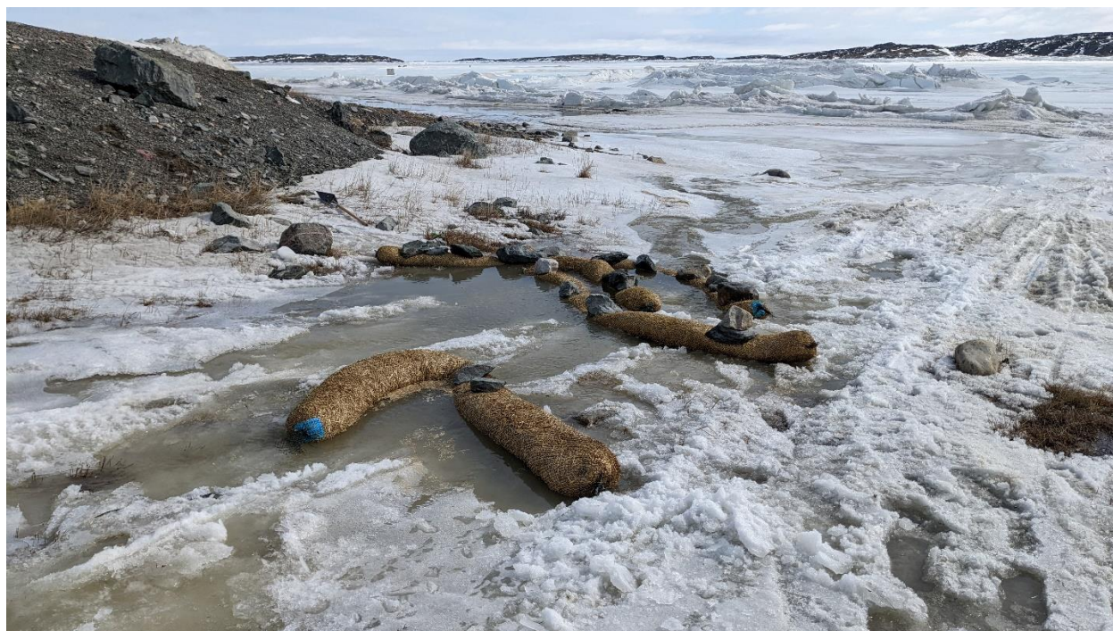
Figure 2: Sediment control at discharge
