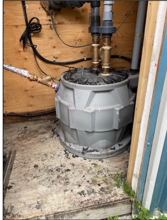
Photo 2: Wing C lift station spill remediation
