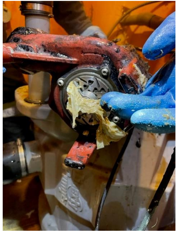
Photo 2: Wing three lift station grind pump blade
