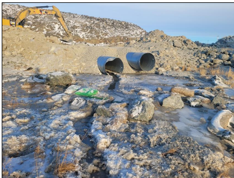
Figure 3: Discharge of pump dewatering downstream of Itivia culverts.
