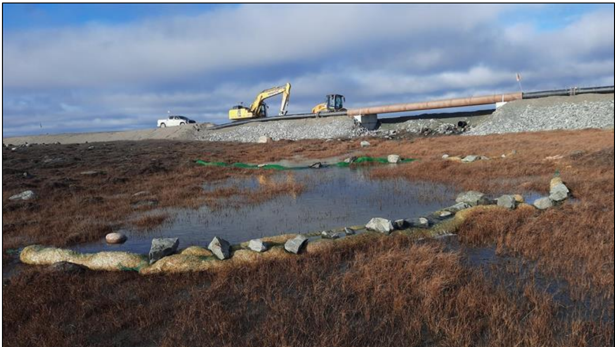
Photo 2: Downstream sediment controls.
