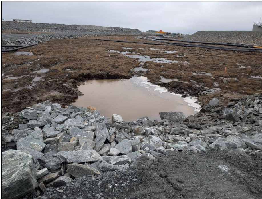
Photo 2: Sump excavated to collect the treated water.
