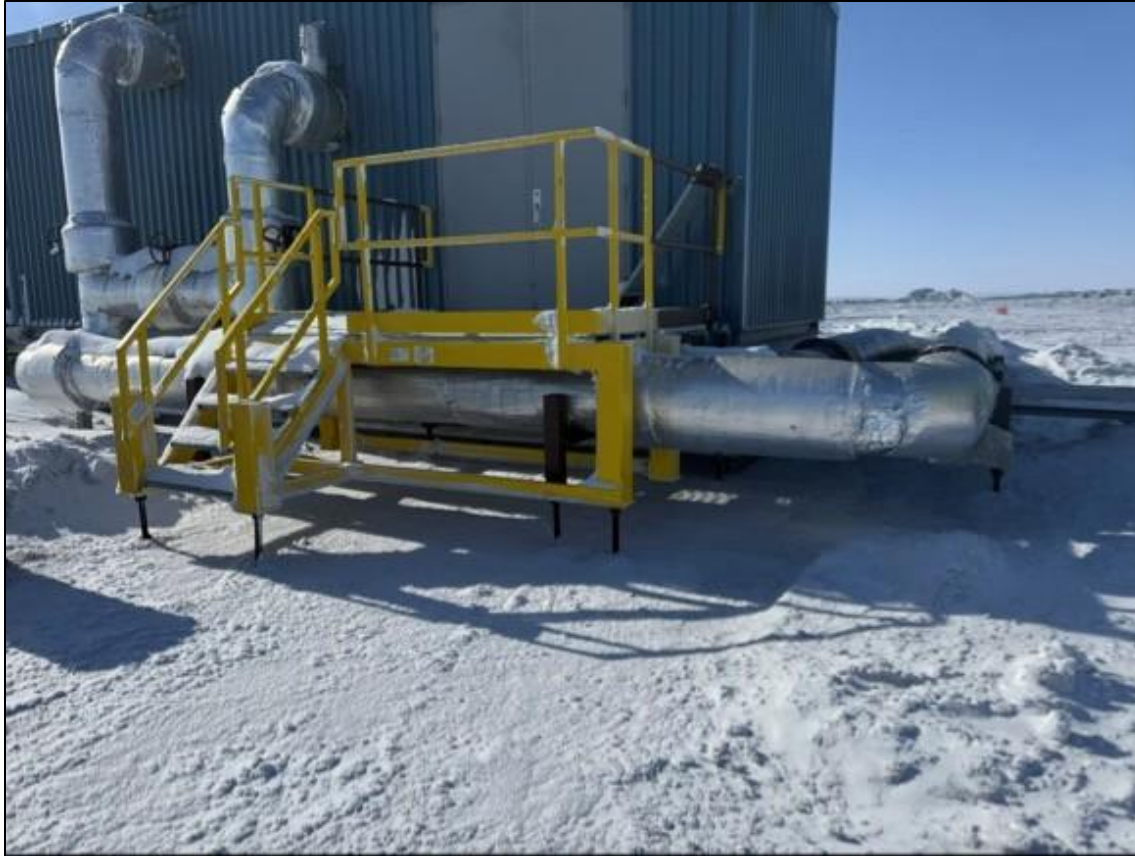
Photo 2: Spill location after remediation.
