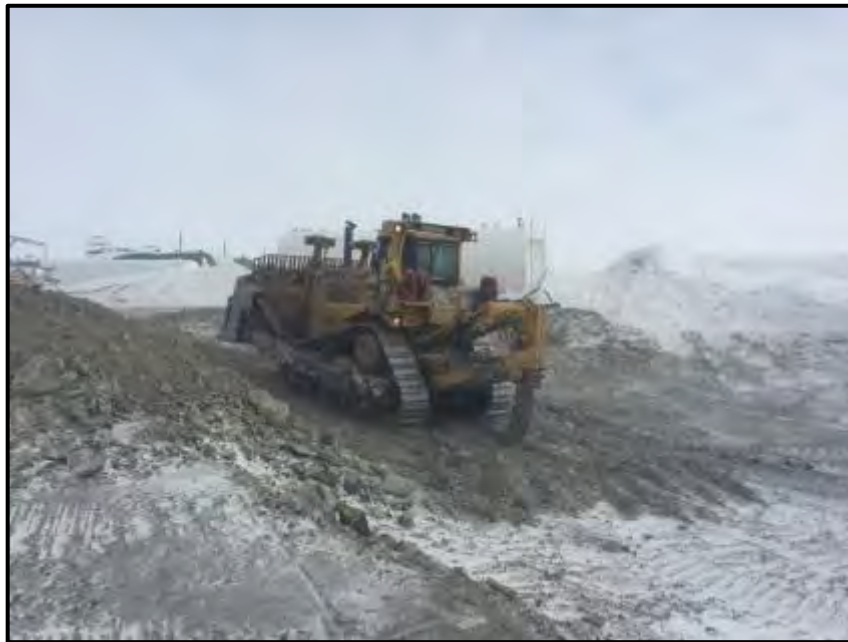
April 17: Removing impacted material from south corner of south excavation.
