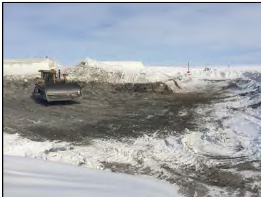
Photograph 20: Ripping north wall of south excavation.
