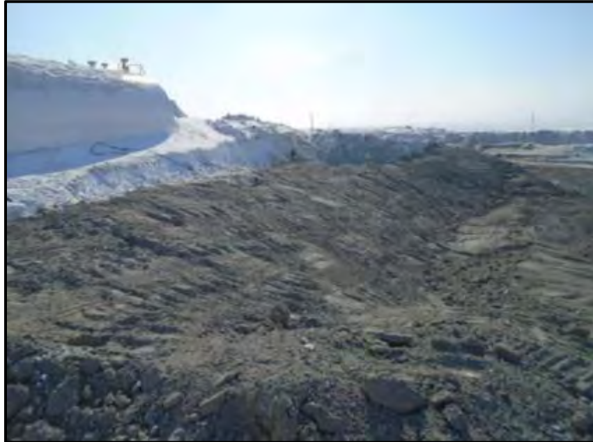
May 2: Backfill material over HDPE liner.
