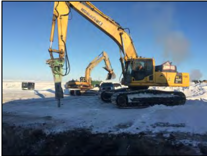
April 15: Hammer and excavator working at approximately 0700hr to remove impacted material from south edge of spill area.
