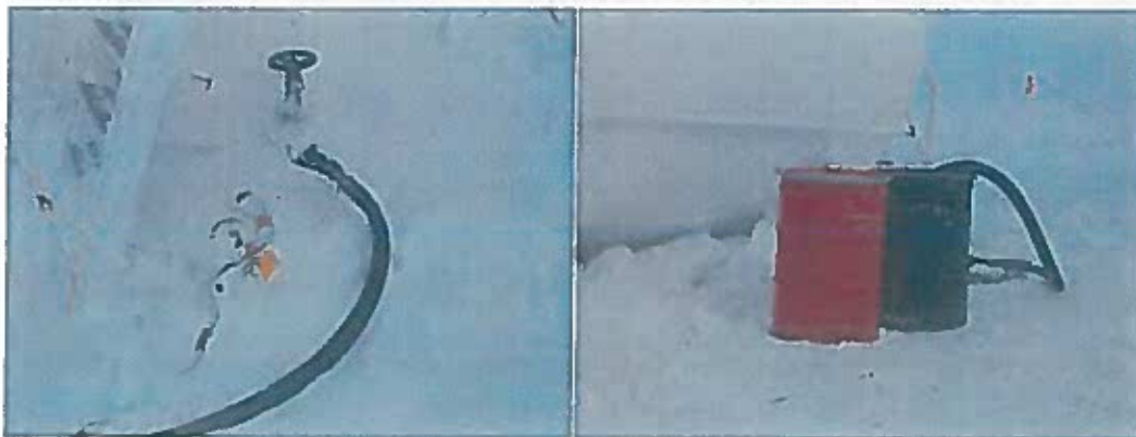
Picture 2: The secondary containment berm underneath the valve is full of contaminated snow – a drum for “fuel contaminated water” has been placed beside the tank for the placement of this contaminated snow
