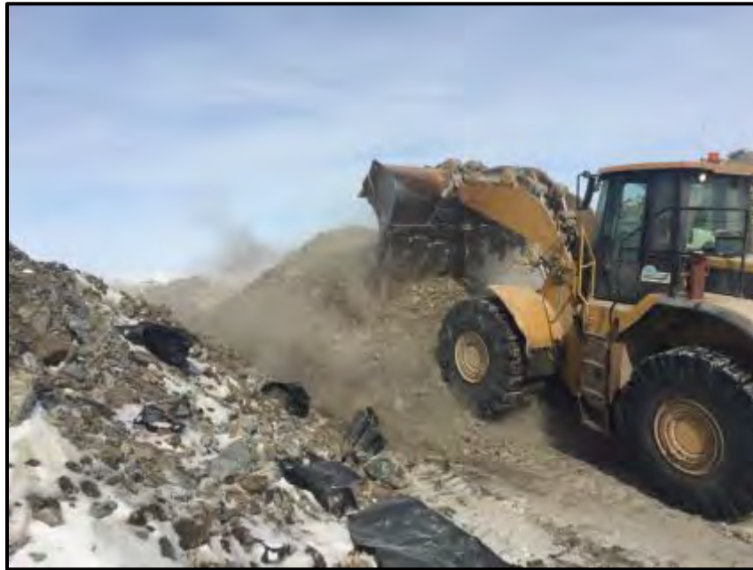
April 20: Dumping contaminated soil in the landfarm.
