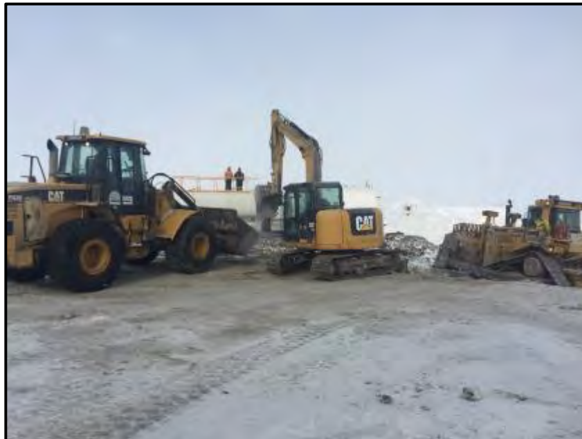
April 17: Taking material to the landfarm with a loader to limit dust from blowing around the site.
