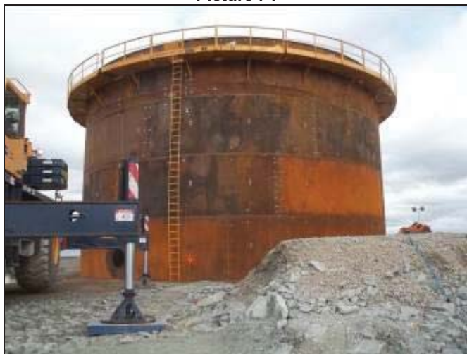
View of tank # 3
