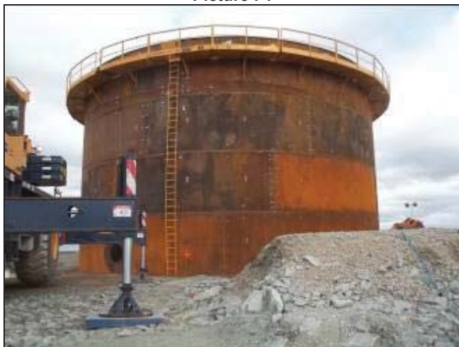
View of tank # 3
