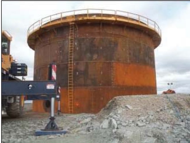
View of tank # 3
