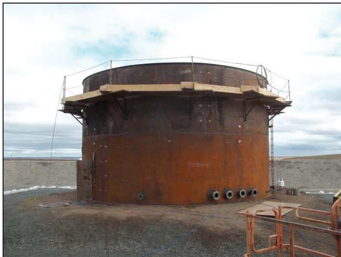
View of tank # 5
