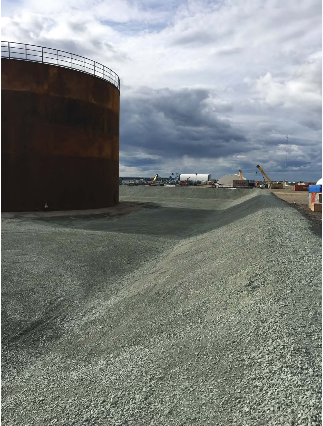
Photo 2 Industrial Site Fuel Farm (view from south-east corner) of secondary containment berm
