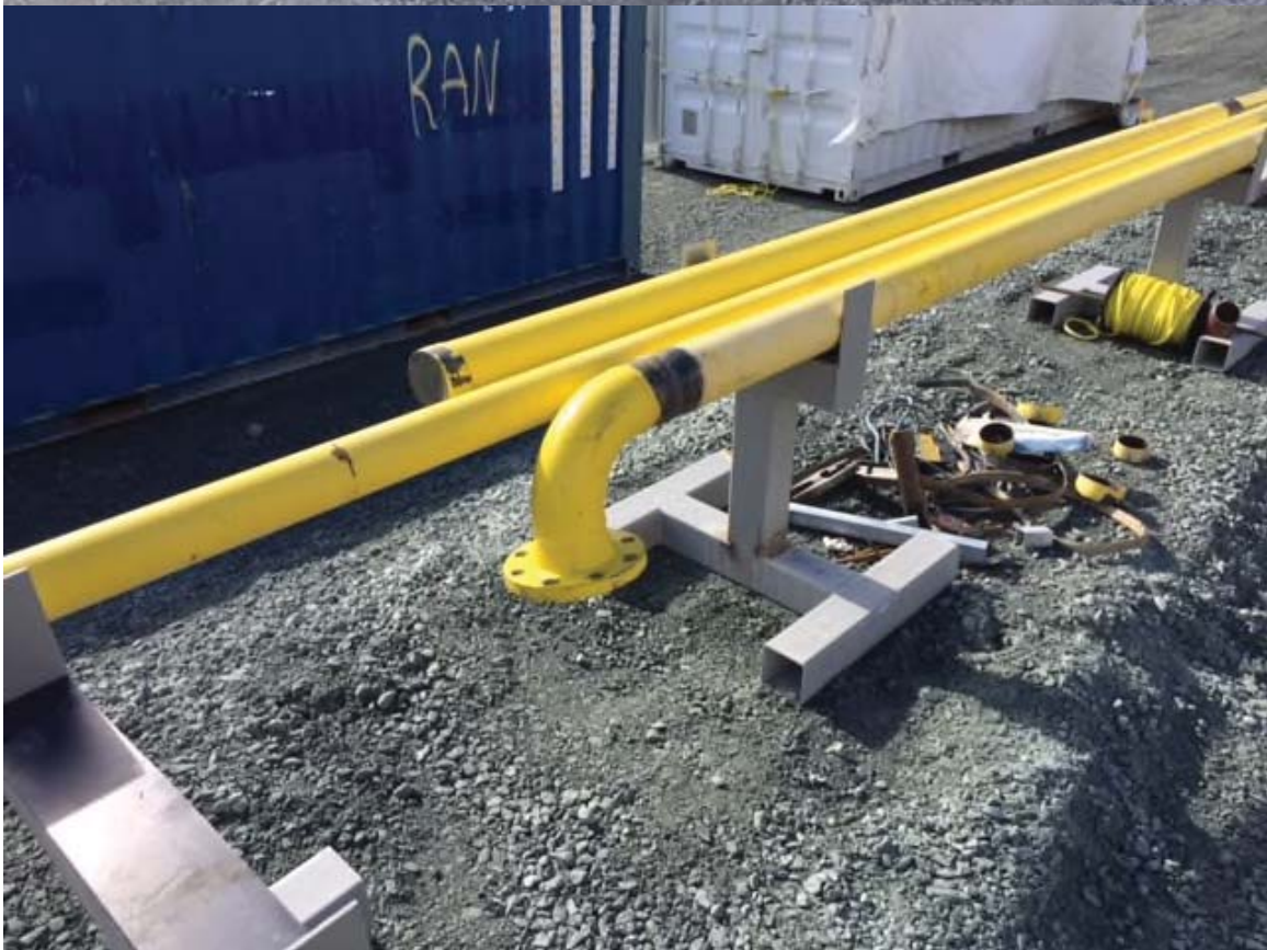
Photo 11 and 12 Pipe support installation
