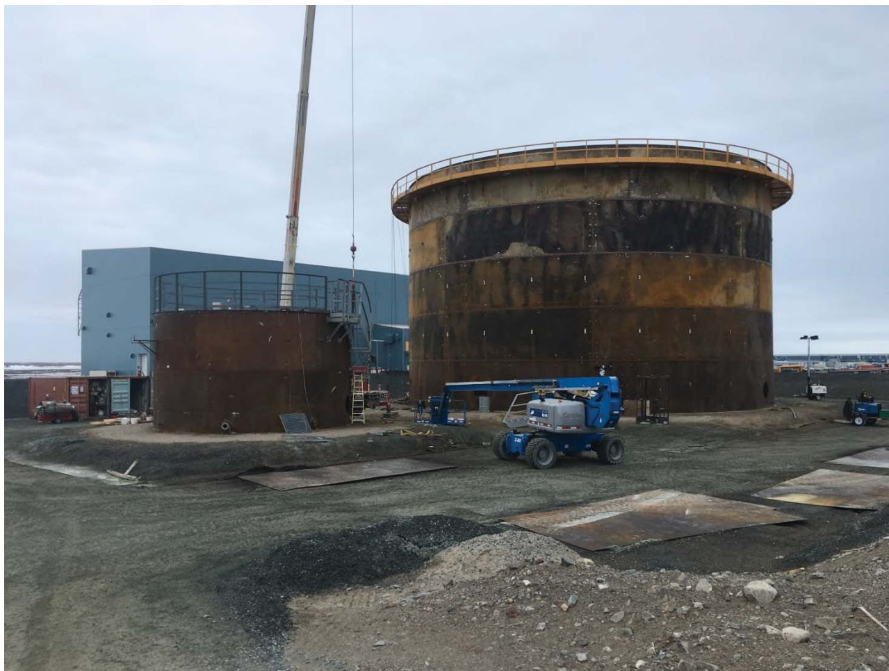
Photo 1 View of Industrial Site Fuel Farm Tank#4 (right) and Tank#5 (left) under construction
