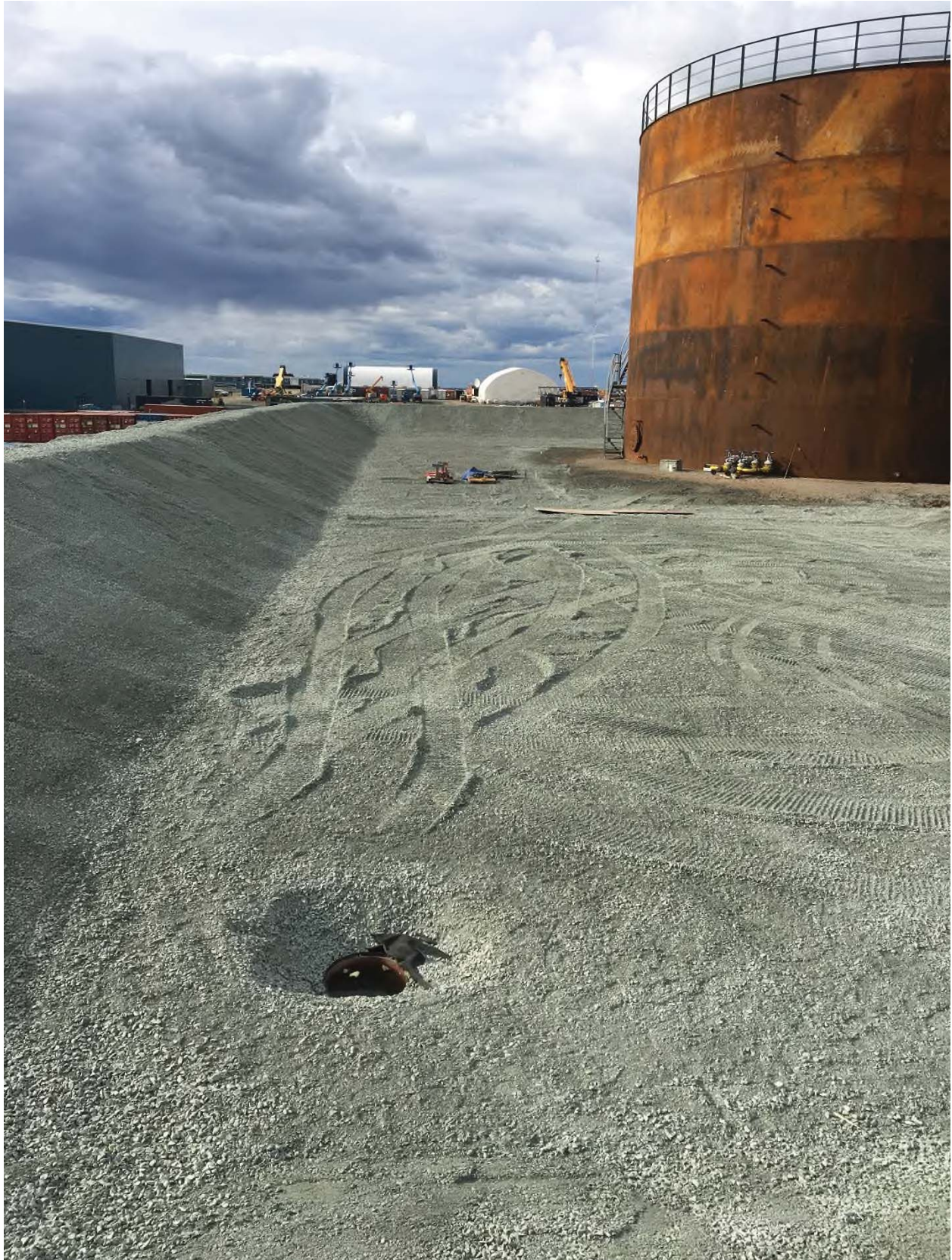
Photo 3 Industrial Site Fuel Farm (view from south-west corner) of secondary containment berm with sump (under construction) in the forefront
