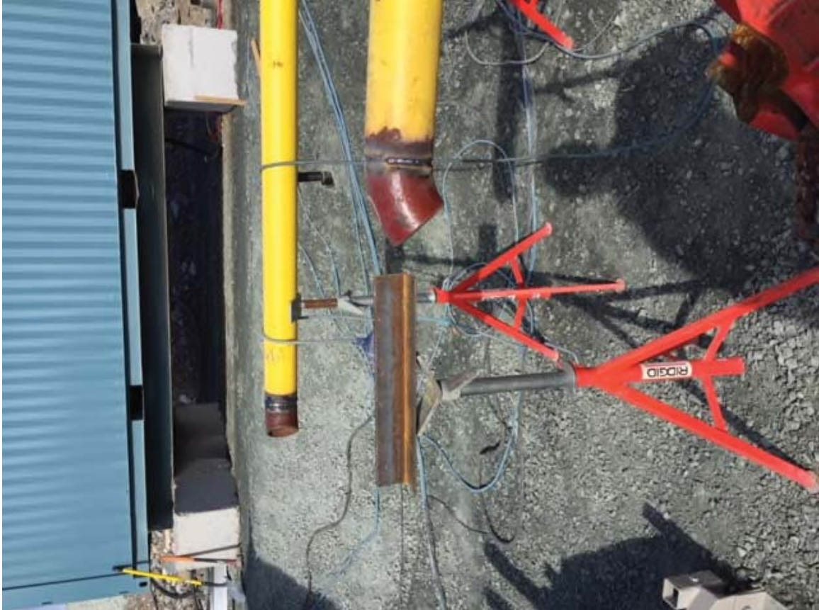
Photos 9 and 10 Welding of pipeline at loading and unloading stations at Industrial Site Fuel Farm
