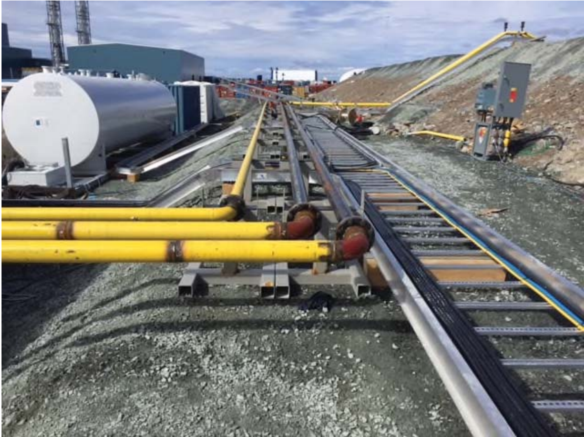
Photo 23 Industrial Site Fuel Farm piping completed
