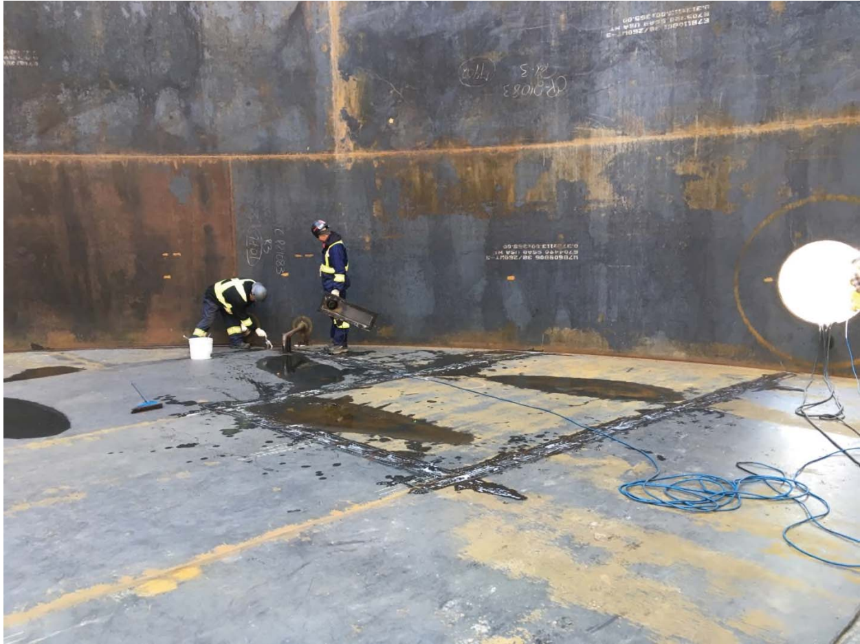
Photo 4 Vacuum tests on floor of Tank#4 (6ML)
