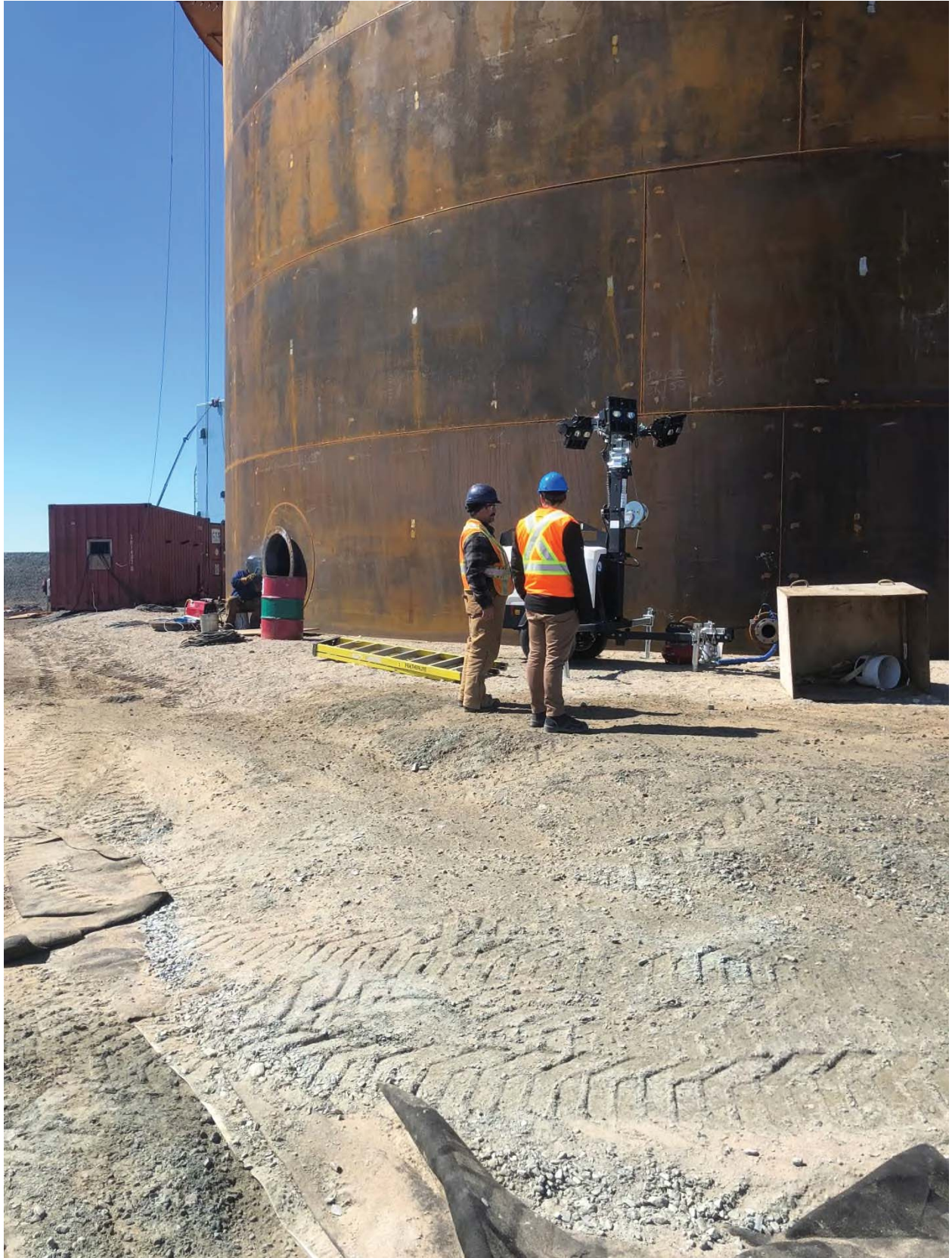
Photo 6 Tank #4 (6ML) looking south
