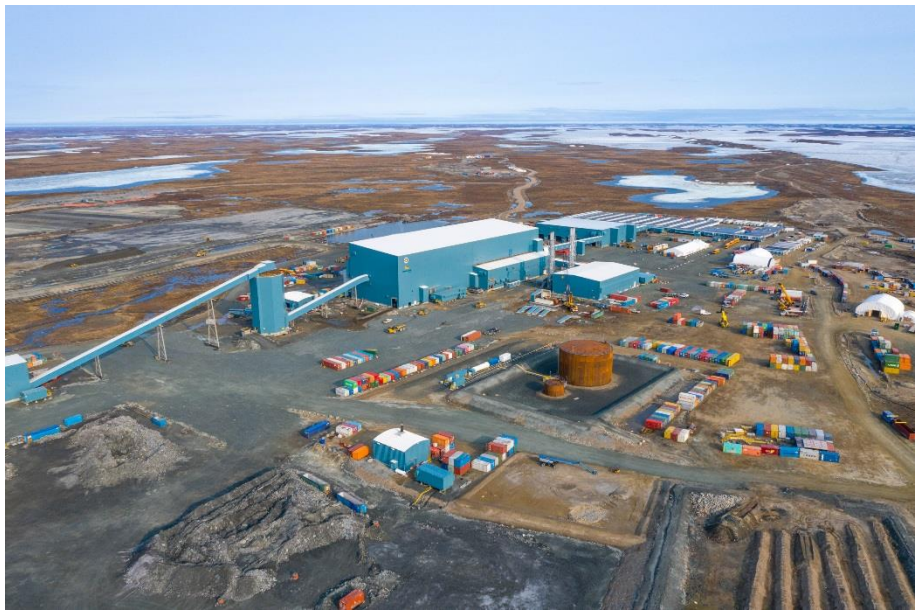
Photo 04: Meliadine site complex, looking northwest (June 2019)
