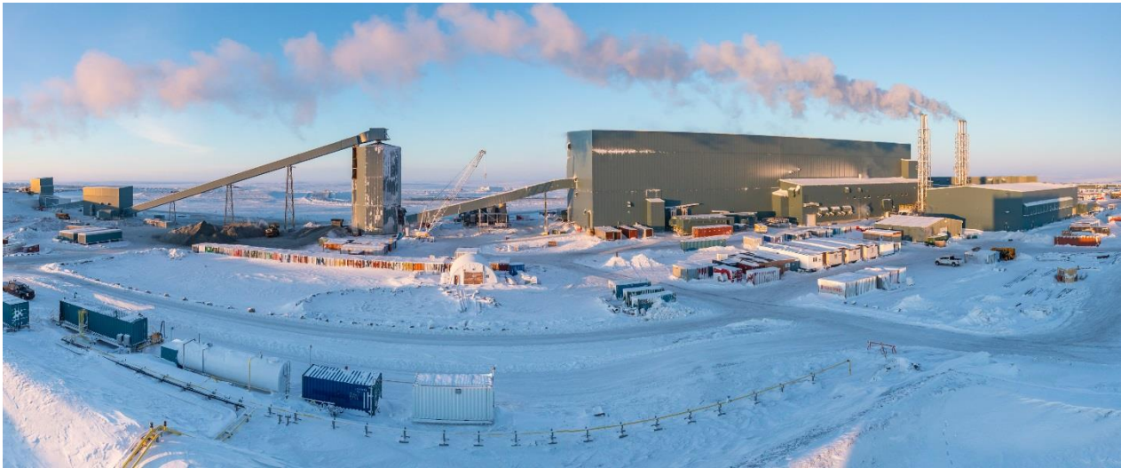
Photo 02: Meliadine Process Facility Complex (February 2019)
