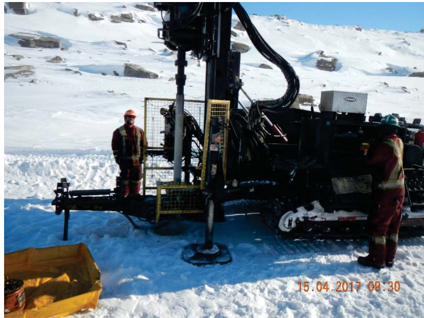
Figure 1: Drilling Rig Setup on a Borehole
