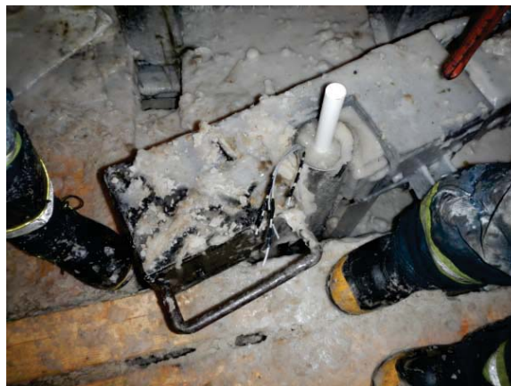
PHOTOGRAPH 3A: Installation of thermistor
