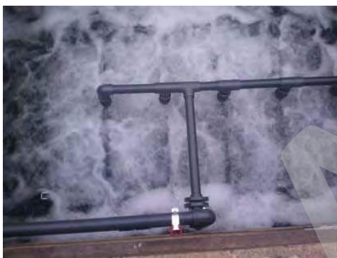
Proper air scouring in membrane tank
