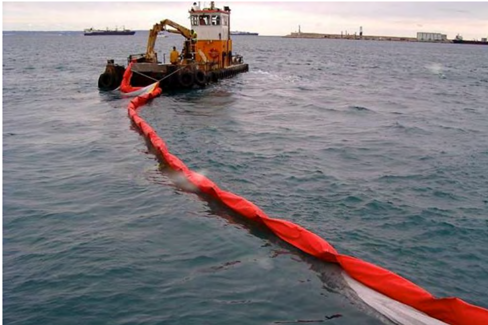
Figure 45: Typical installation of a silt curtain
