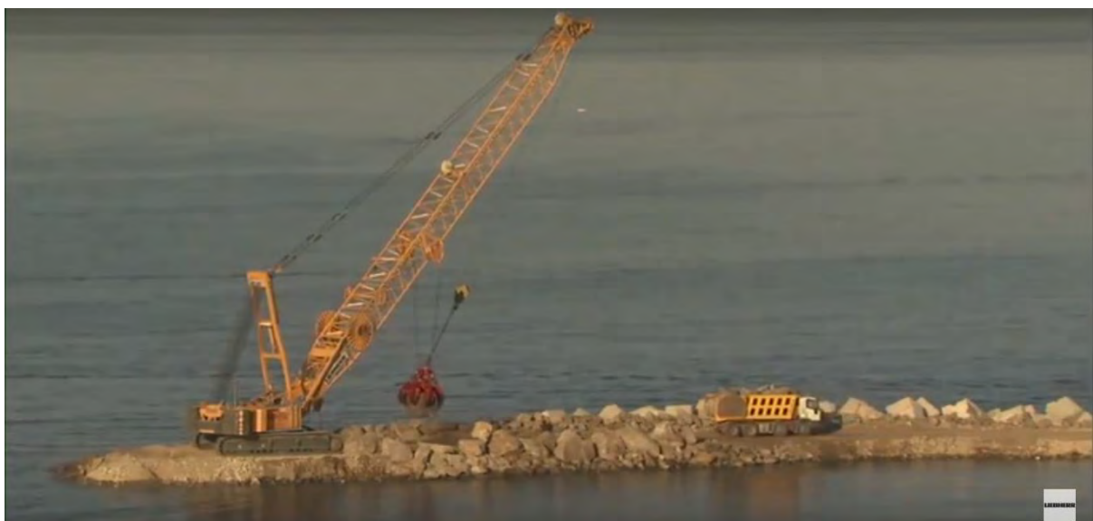
Figure 21: Armour rock placing with crane and hydraulic grab
