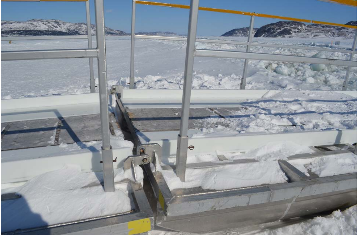
Figure 5 The Connection Points Between Units.
