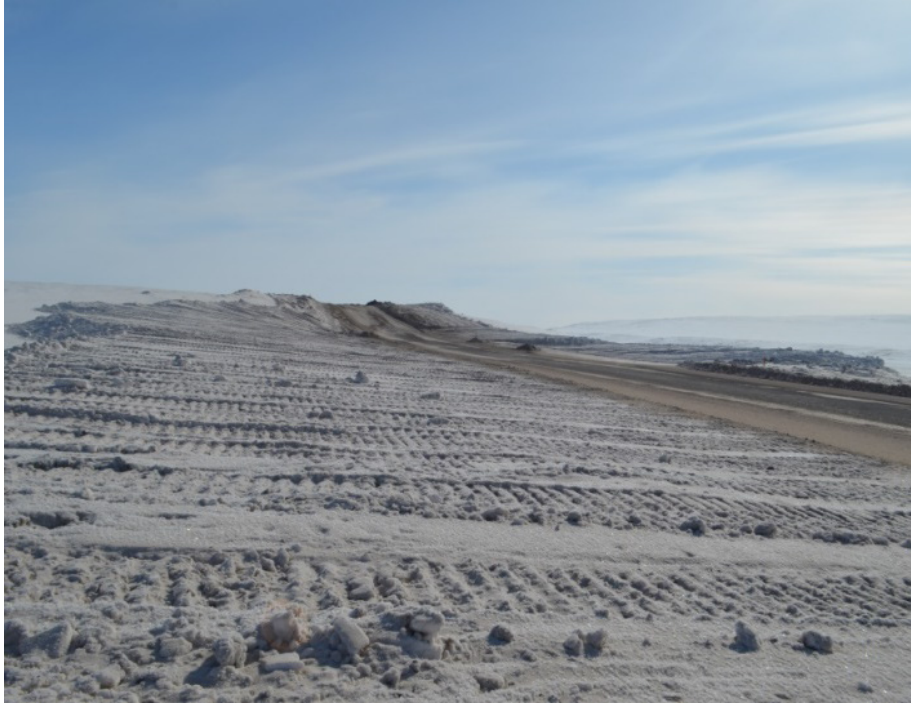
Photo 1. Example of snowbank management on east and west sides of Tote Road to reduce snow drifting and confirm that snowbanks do not exceed the maximum snow depth (km 28, April 21, 2017).
