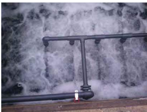
Proper air scouring in membrane tank
