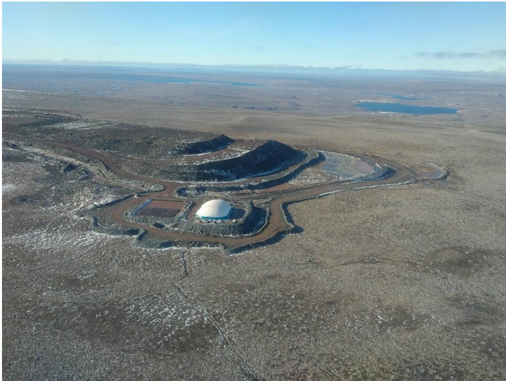
Waste Rock Facility, facing northeast
