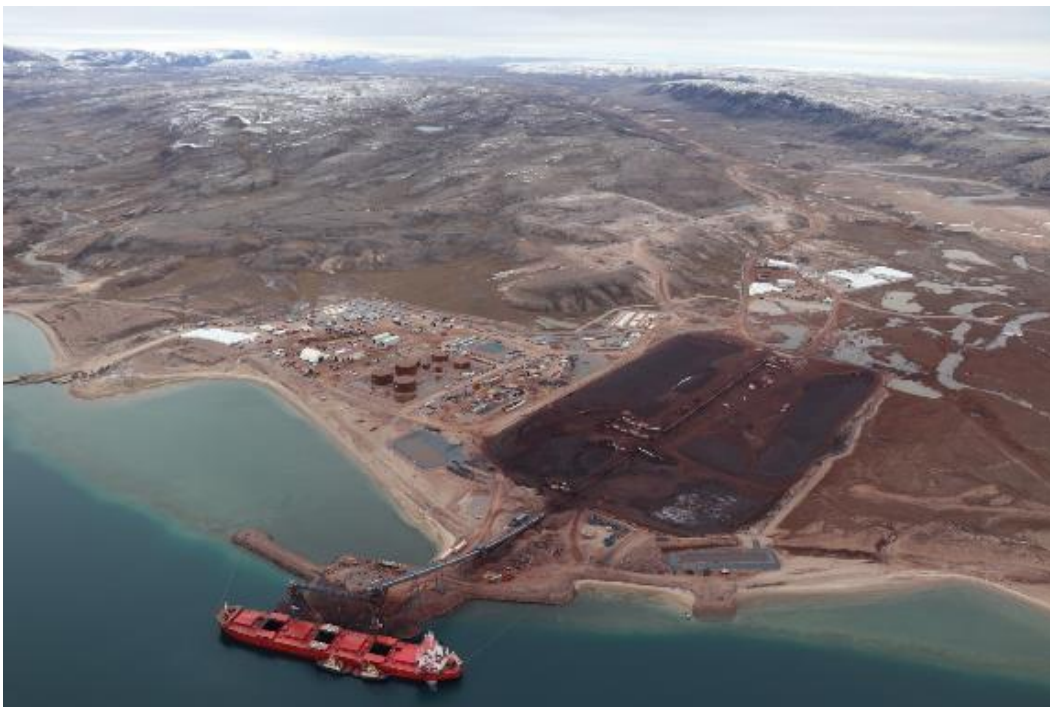
Milne Port – View Southeast
