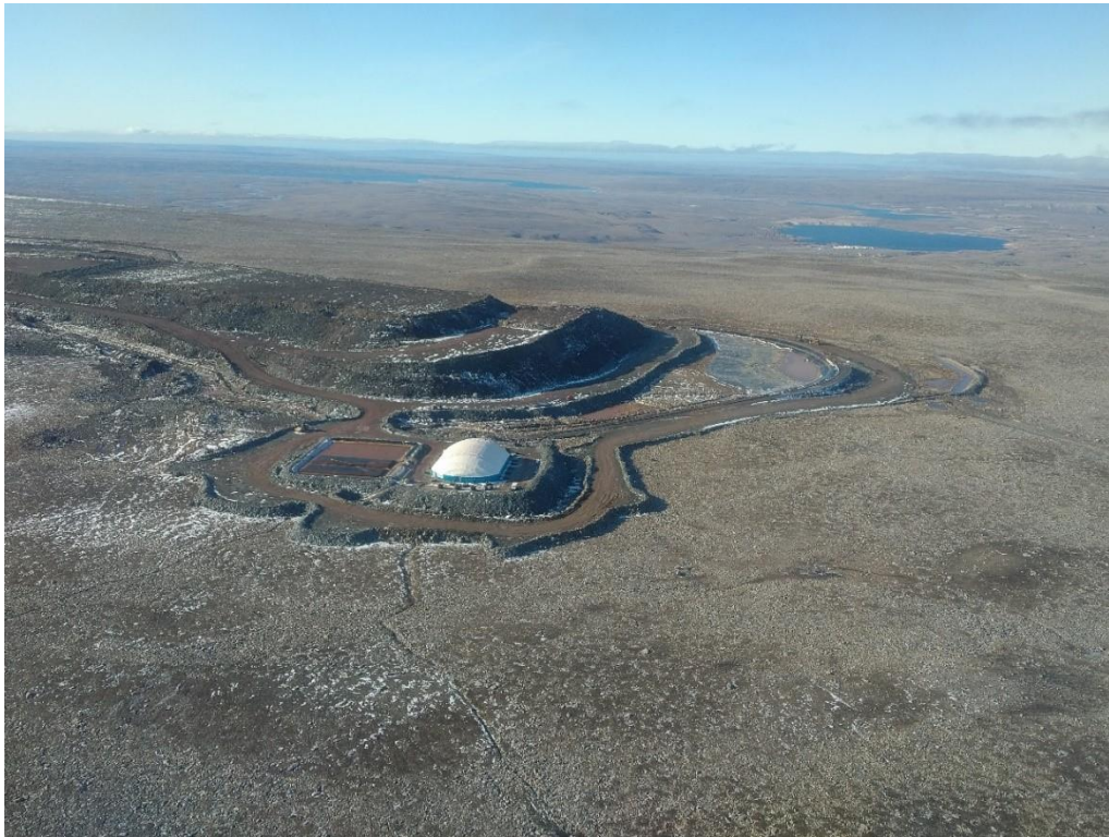
Waste Rock Facility, facing northeast
