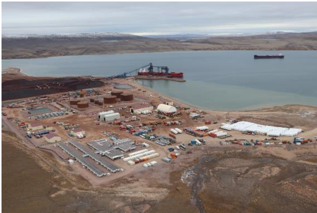
Milne Port – View Northwest
