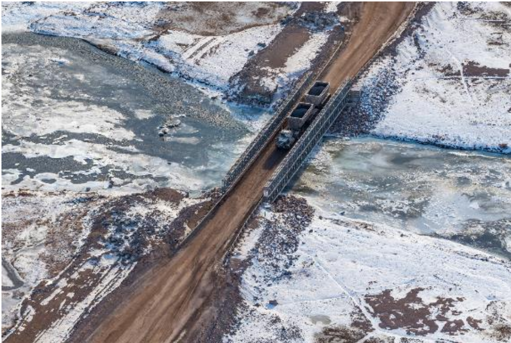
Tote Road Water Crossing
