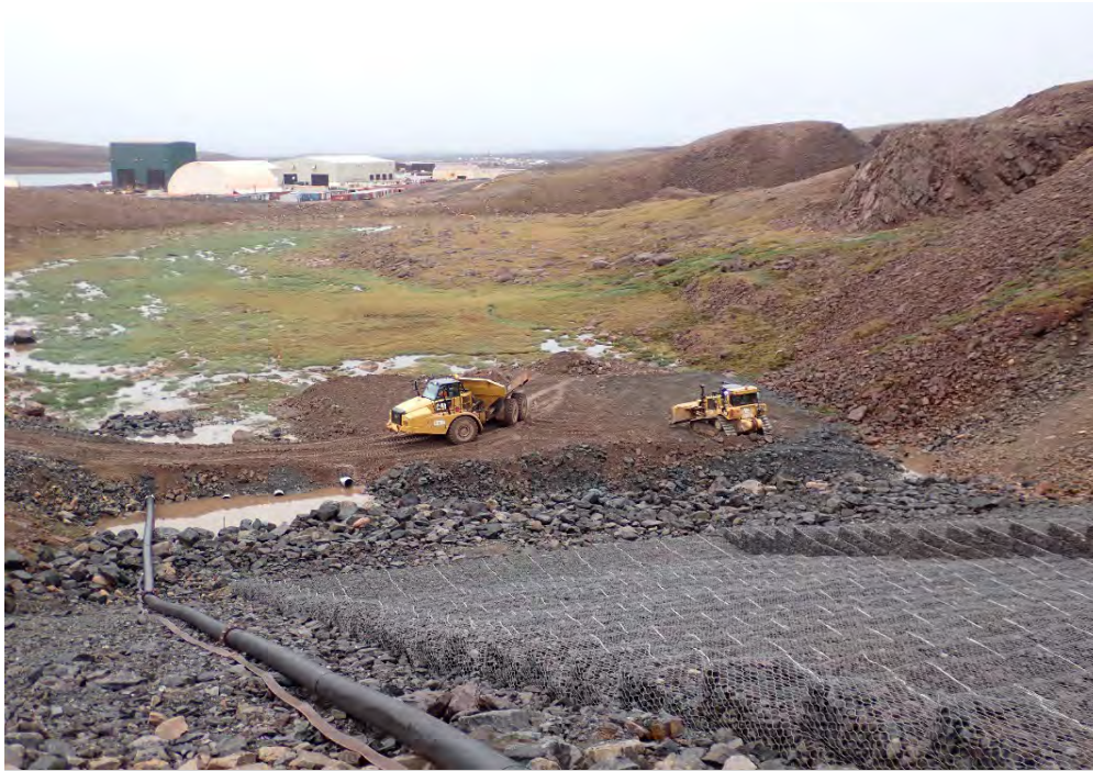
Photo 40 – Construction of Geotube Pad at Mine Site KM105 Surface Water Management Pond (MS-11) – August 2023
