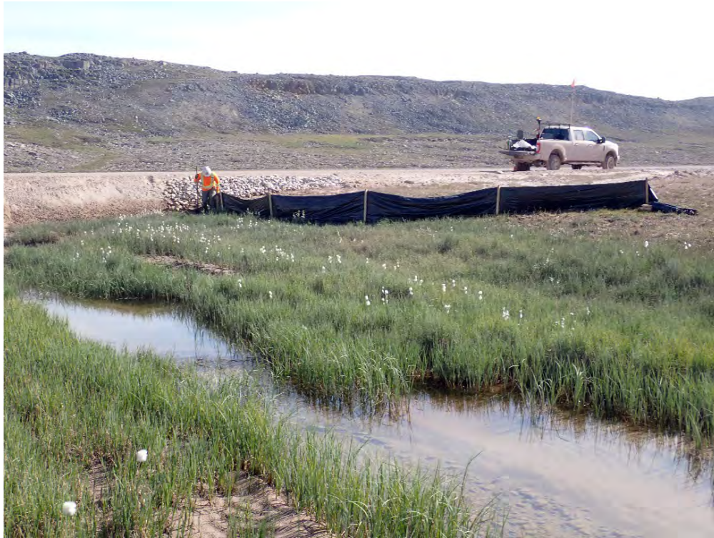
Photo 86 – ESC Installation – August 2023
