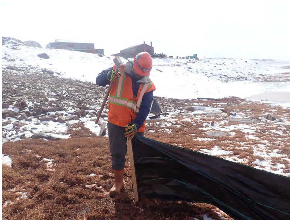
Photo 87 – ESC Installation Upstream of CV-187 – June 2023
