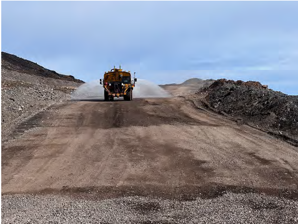
Photo 93 – Mine Haul Road Dust Suppression – July 2023
