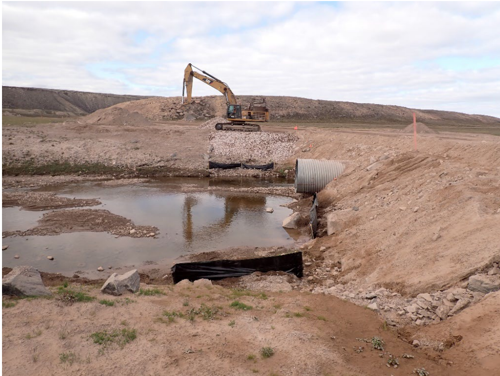
Photo 41 – Installation of Ditch Armouring, Check Dams, and Silt Fencing at KM94 – July 2023
