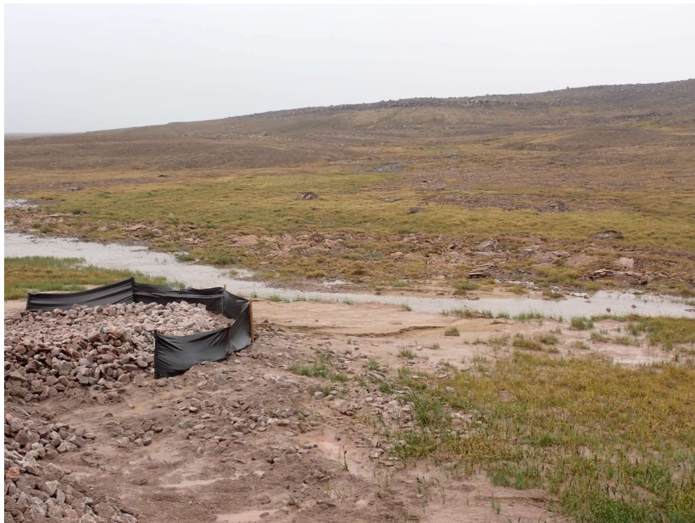
Photo 40 – Swale reinforced with armor stone and Silt Fence Installation at KM 53 – August 2023
