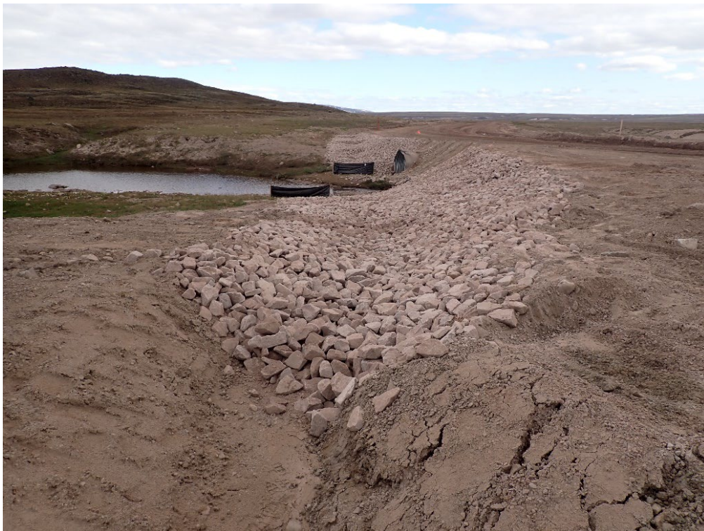
Photo 42 – Installation of Ditch Armouring, Check Dams, and Silt Fencing at KM94 – July 2023
