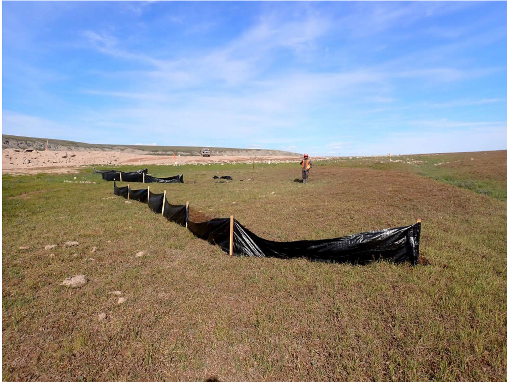
Photo 39 – Silt Fence Installation at KM 75– August 2023
