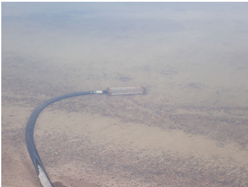
Photo 28 – Installation of End-of-Pipe Fish Screen at KM80 – July 2023
