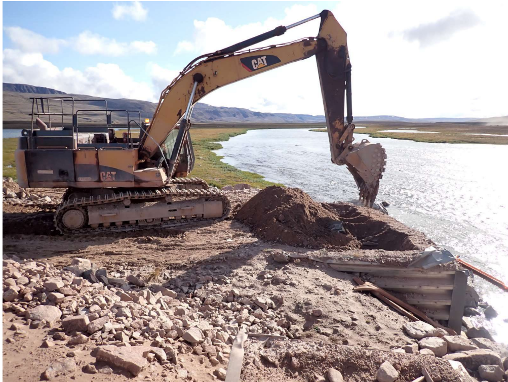
Photo 13 – Excavator removing old KM17 Bridge Abutment with Silt Curtain in place– August 2023
