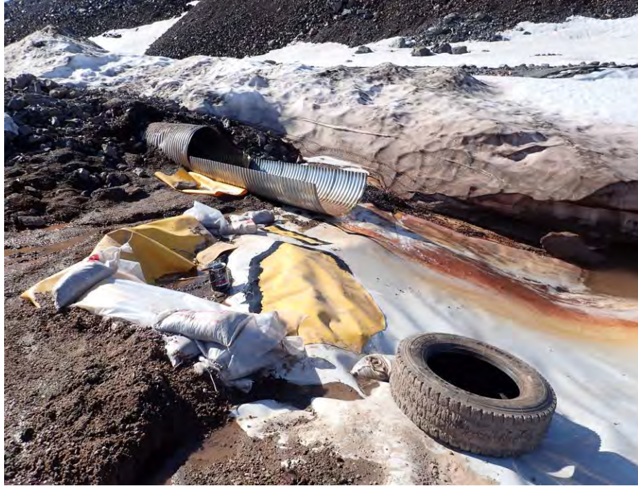
Photo 1 – Liner repair at the WRF pond ditch inflow. July 16, 2023
