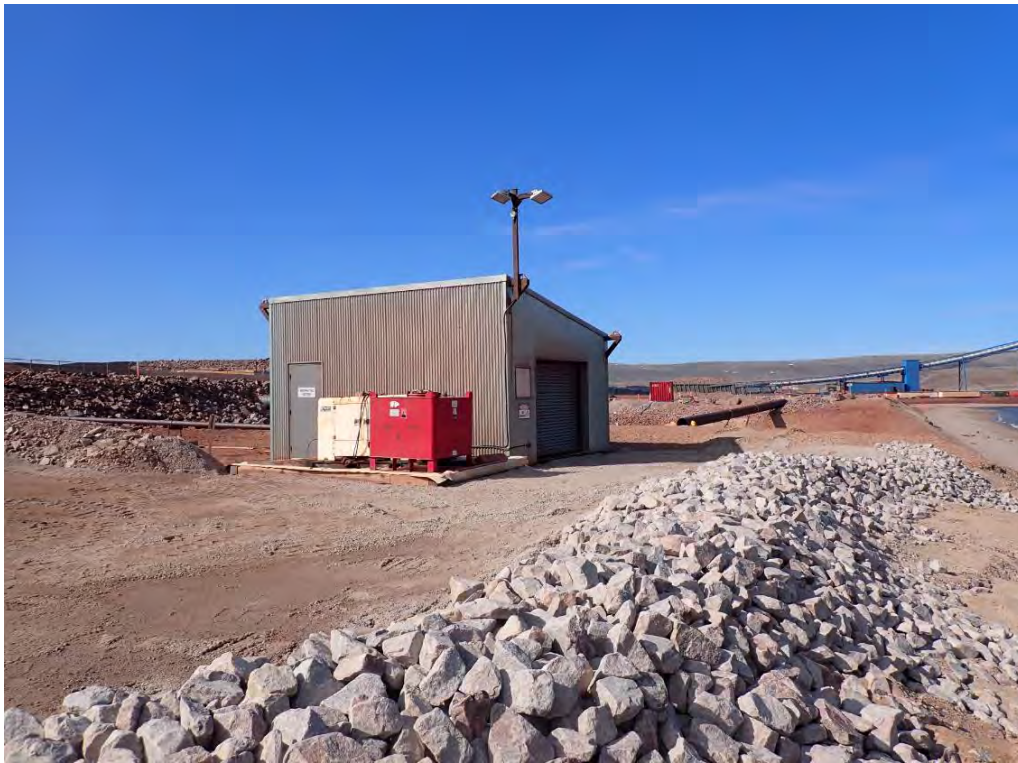
Photo 6 – Follow up to spill 23-294 showing re-enforced bank to prevent further erosion
