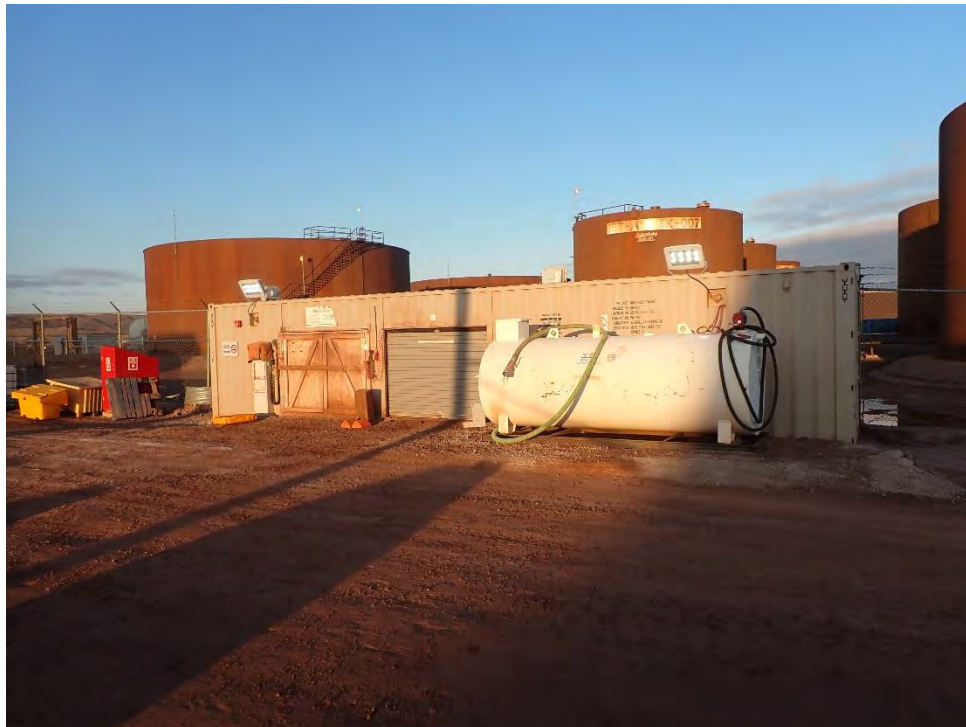
Photo 4 – Contaminated soil removed, and old fuel tank replaced with new double walled tank. September, 2023
