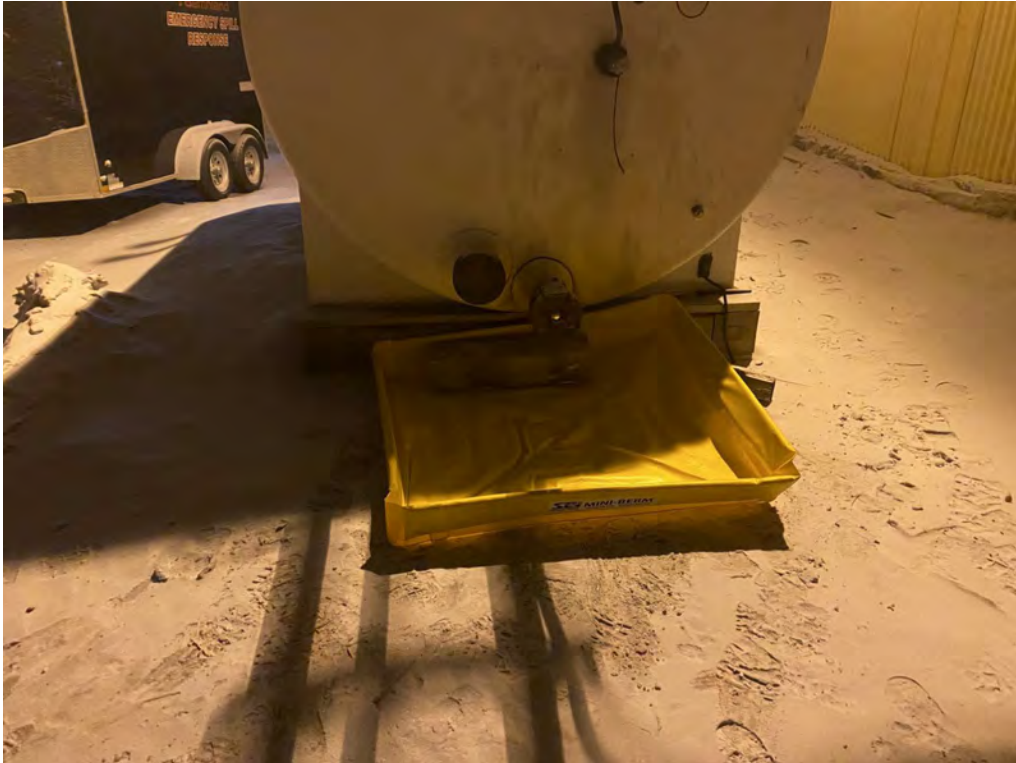
Photo 2. Fuel Tank at Mine Rescue Building after Valve Repair (with Temporary Spill Tray), Feb 13
