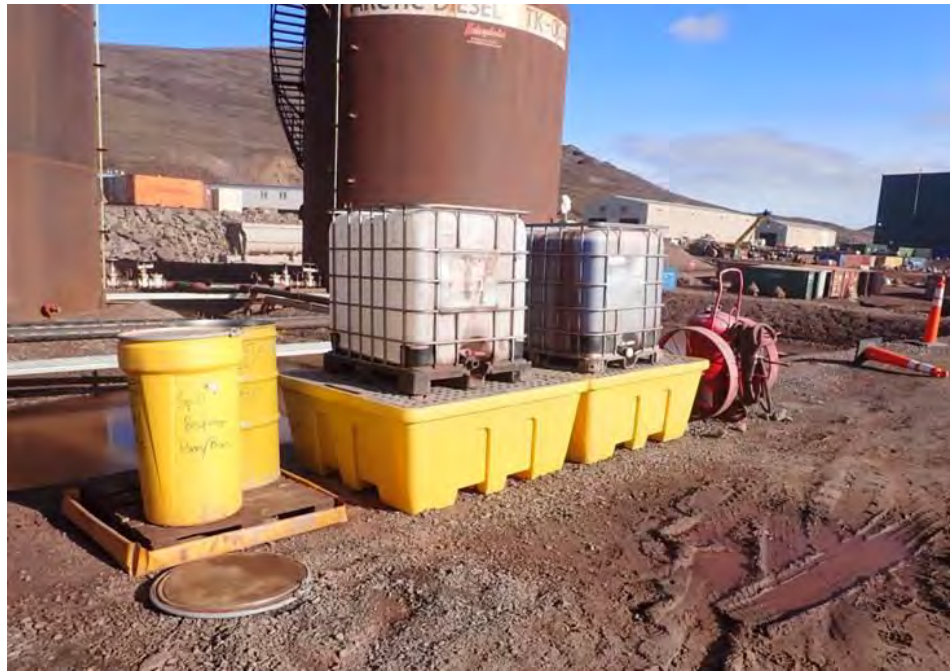
Photo 3 – Spill trays at Mary River light vehicle refueling area replaced, August 2023
