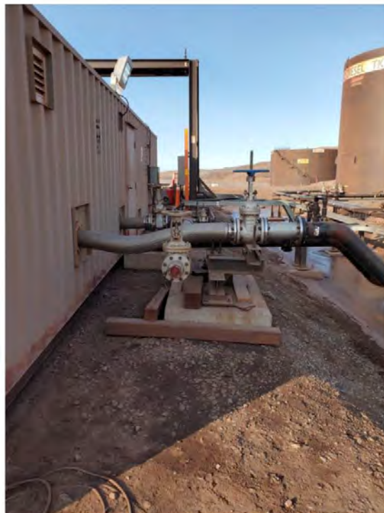
Photo 2. Mary River fuel filling station showing stained substrate removed under flex line. Sept 16, 2023
