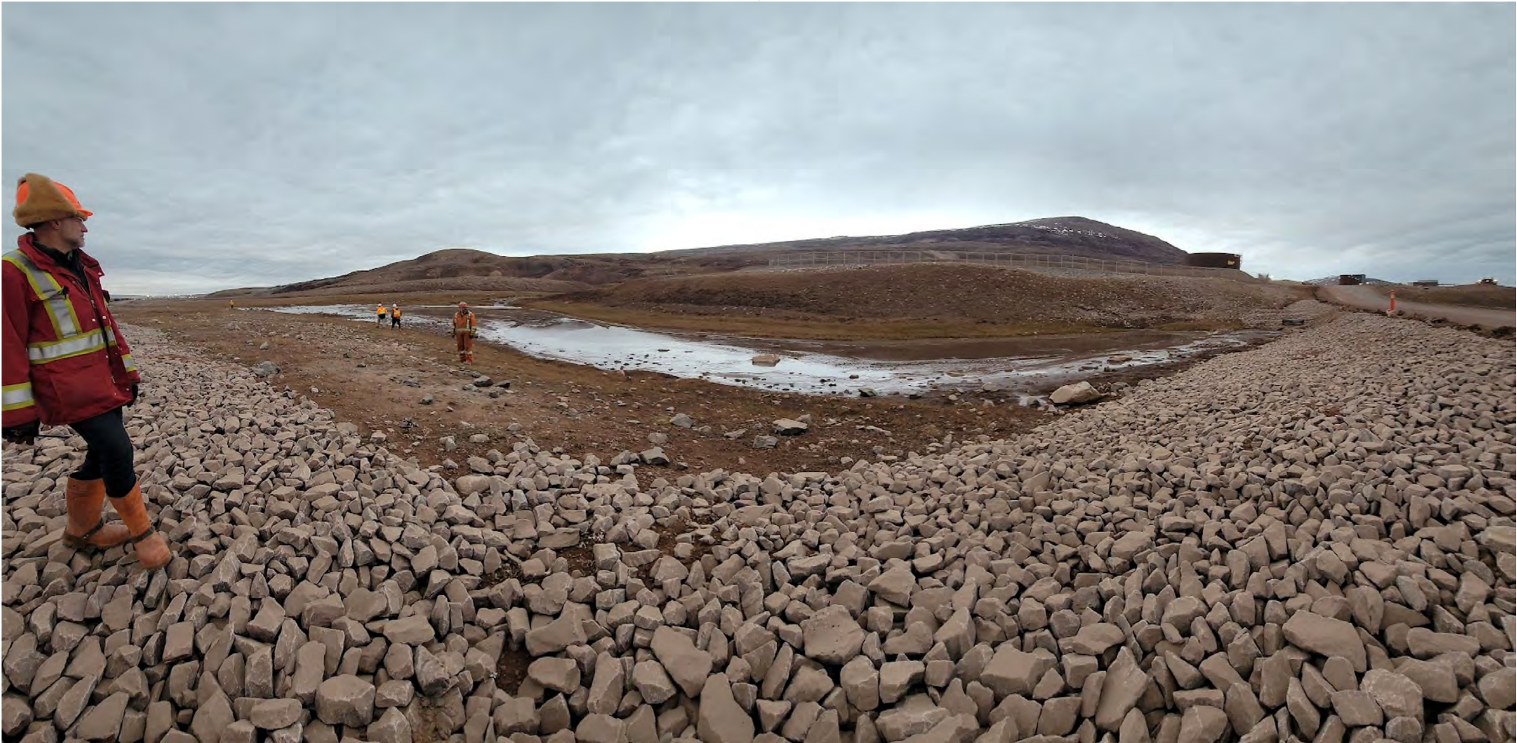
Photo 10B: View of north side of Tote Road just east of Sailivik Camp where armoring and sediment control civil works were completed in the period between the two independent environmental Inspections completed in 2023.
