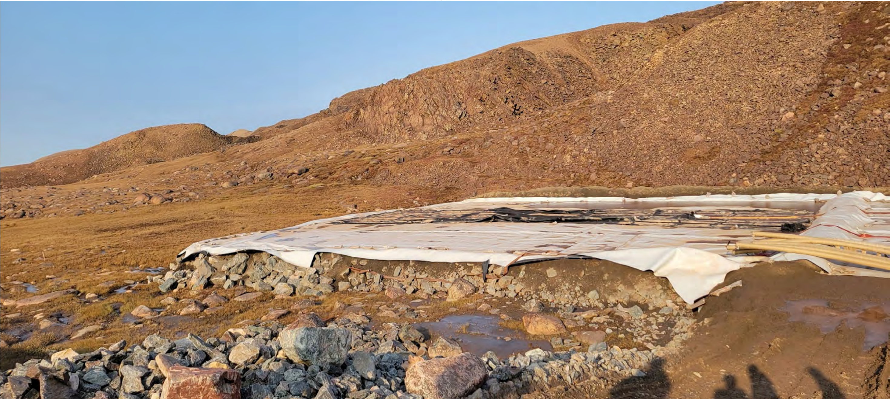
Photo 7: View of pad extended northwards and adjacent to the downstream toe of the KM 105 Northwest Embankment. The black geobag (pictured) lies on top of a white geomembrane. At the time of the September 2023 Inspection, the geobag was not in use. Site personnel indicated that the system was installed at some point after the June 2023 Inspection to capture sediment laden water seeping from the toe of the embankment. It is recommended that this system be configured to provide an auxiliary line of defense to mitigate undesirable sediment loading to waters that ultimate report to Shear Down Lake. It was also noted that the pad created was extended beyond the original limits expected by QIA. A technical memo should summarize and provide details about the installation.
