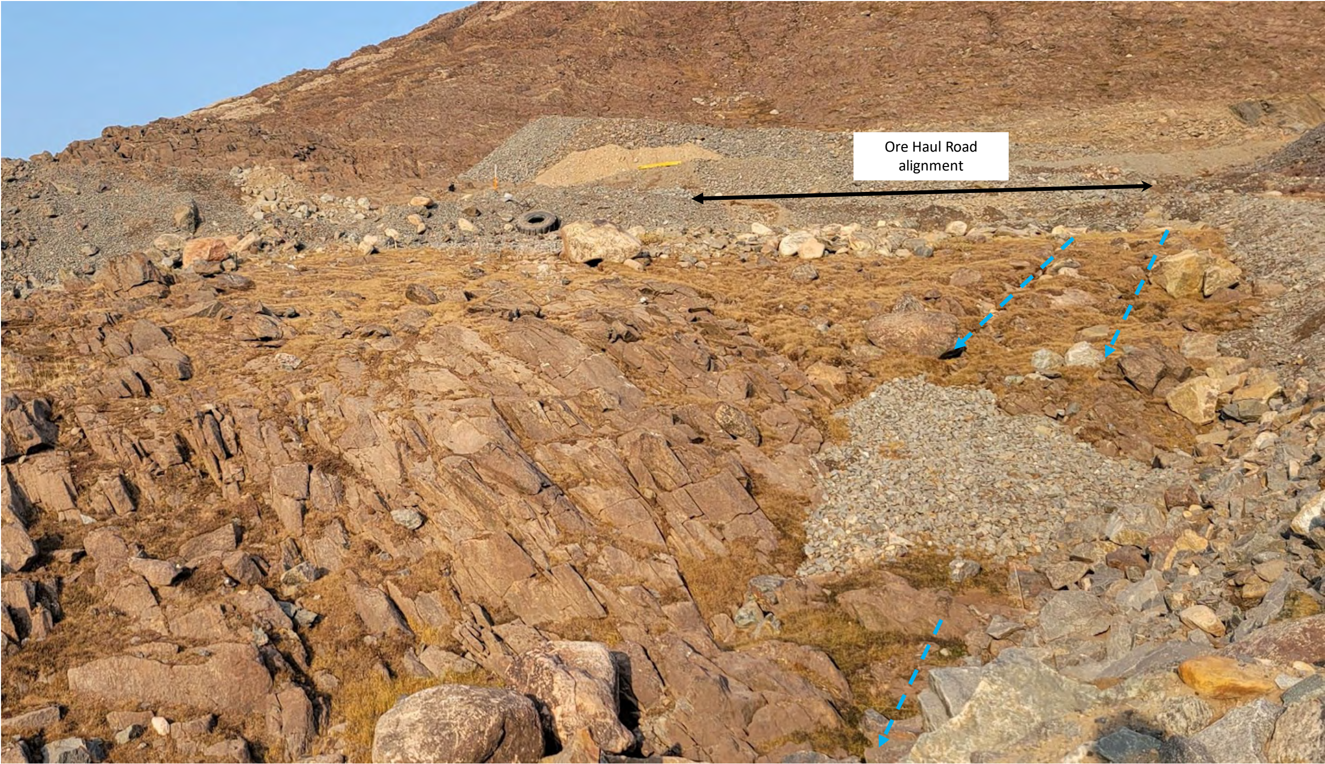
Photo 3: Area south and west of the southwest corner of the KM 106 Ore Stockpile with open geological structure that appears to allow water to flow through. Direction of water flow is shown.
