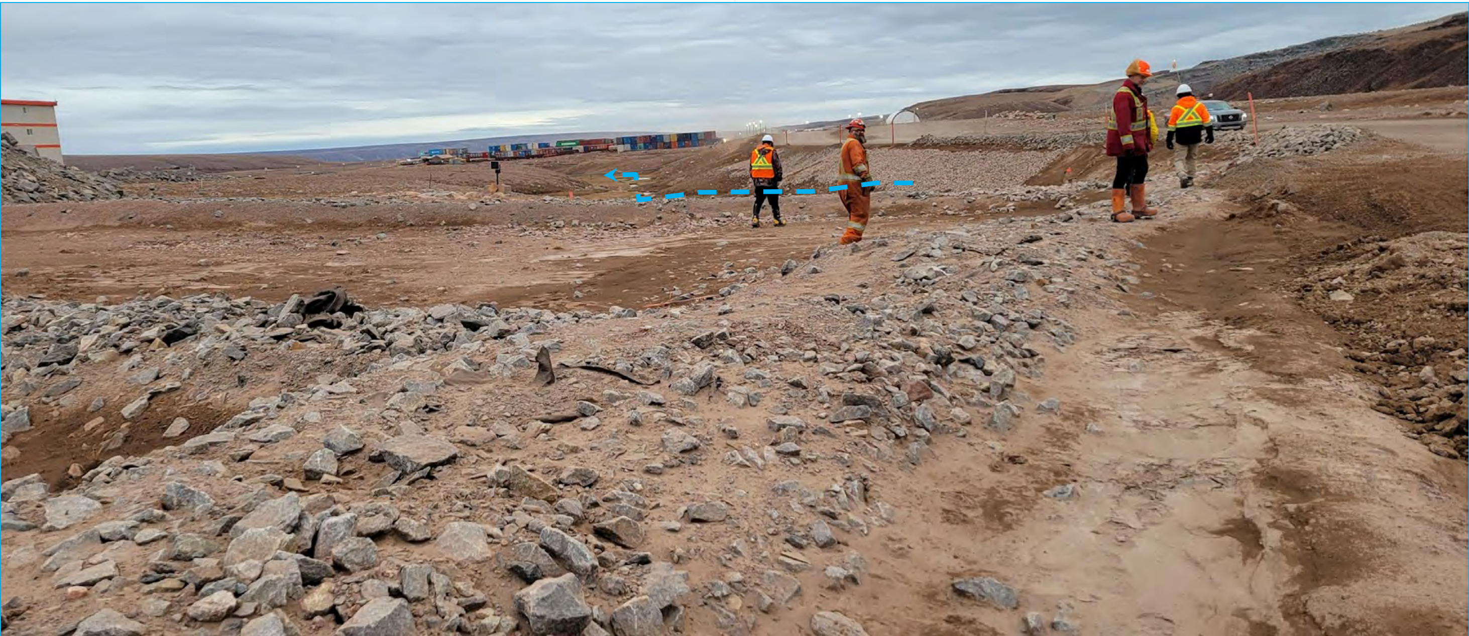
Photo 11A: View of riprap covered in sediment upstream of the channel that convey water to Sheardown Lake. Annual maintenance should include removal of accumulated sediment to allow sediment control structures to work effectively during the annual freshet. The broken blue arrow shows the direction and flow path of the water course that heads towards Sheardown Lake. This area is located north of Sallivik Camp but on the south side of the Tote Road. View looking northwest towards the laydown area.
