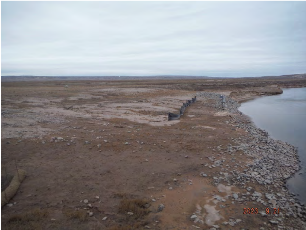
Photo 13 – km80 watercourse crossing where ESC measures have been implemented (Sep 2023).
