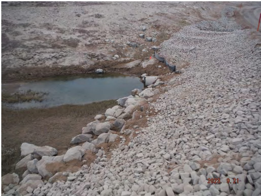
Photo 12 – Km85 watercourse crossing where erosion control with rock has taken place (Sep 2023).
