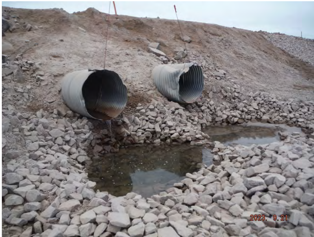
Photo 9 –SDCT-1 Tributary at km63 perched culverts (Sep 2023).
