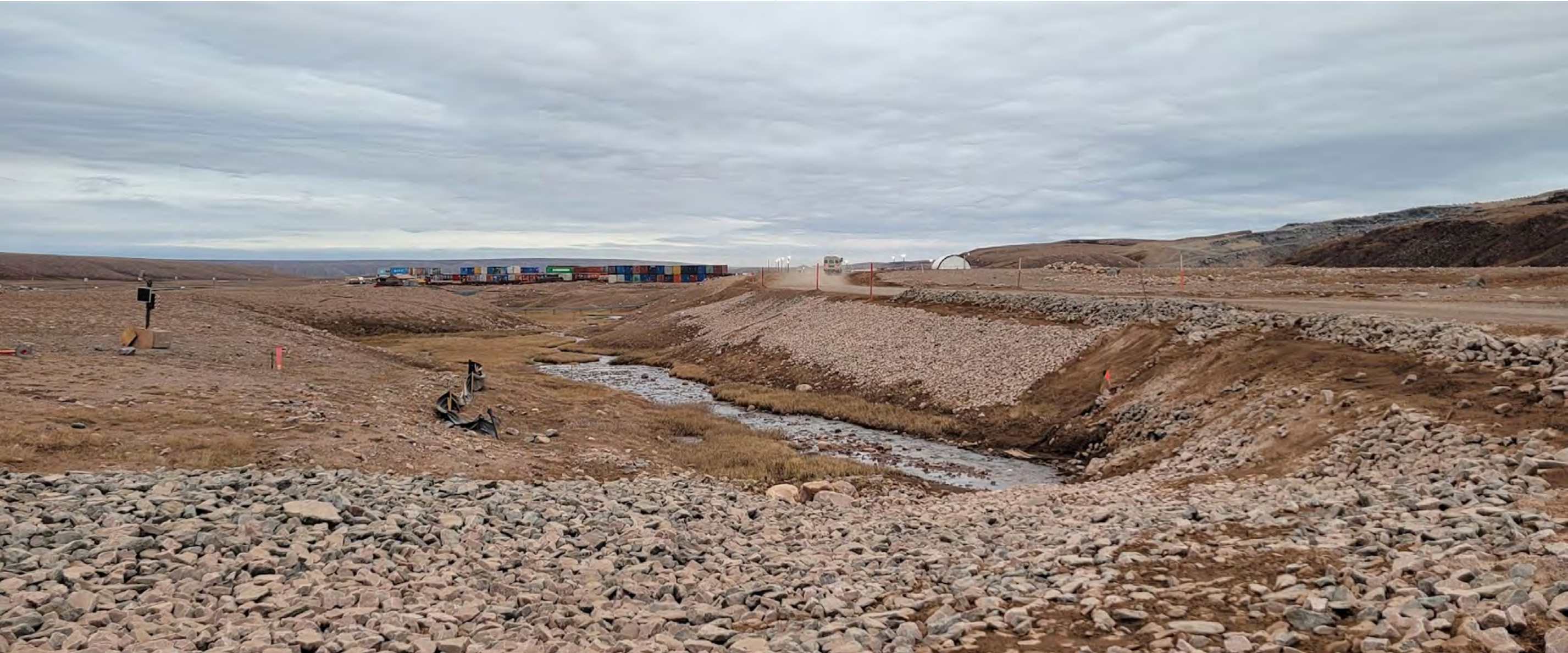
Photo 11B: Closer view of side slope armoring upstream of channel conveying water to Sheardown Lake pictured in Photo 11A. Areas of accumulated sediment on the surface of rock armoring are evident and in need of cleaning prior to the onset of the 2023 freshet. A commonly observed condition of silt fences at the site where they have been installed is also seen left of the center of the photo. It is recommended that silt fences be replaced by coir logs which have improved filter and sediment capture capability with the added benefit of greater durability, especially in this application context.
