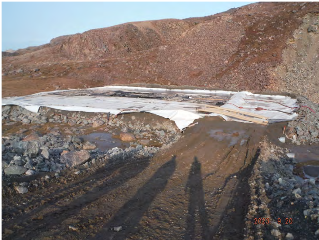
Photo 2 – Geobag downstream of dam/pond at km105 (Sep 2023).
