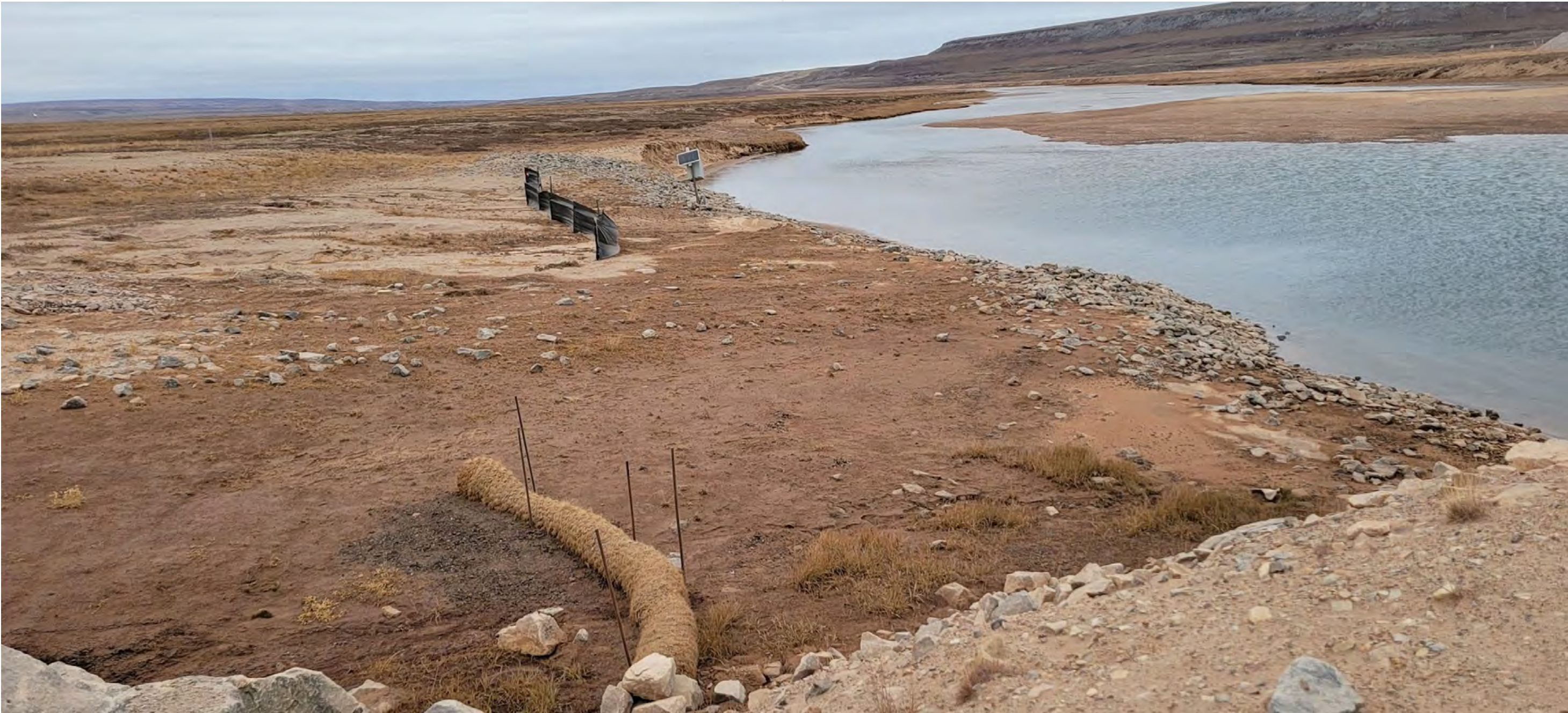
Photo 12: View of areas on south bank of river at KM 80 crossing showing use of both a silt fence and a coconut coir log. This area should be monitored to ensure that sediment control measures work as desired and adequately mitigate sediment runoff into the adjacent water body.
