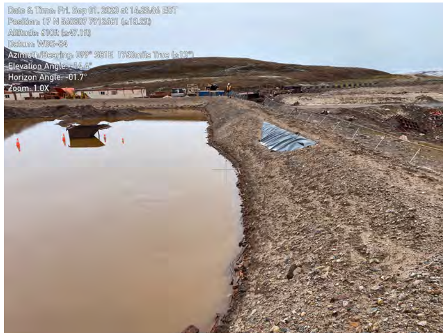
Figure 3.7: Exposed geosynthetic liner on inside of Landfarm berm.
