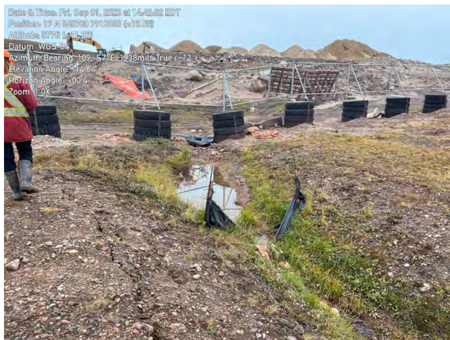
Figure 3.8: Uncontrolled runoff from landfill to surrounding environment.
