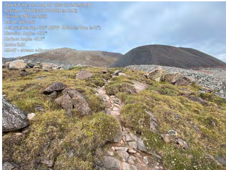
Figure 3.3: Seepage path bypassing MS-07 sediment pond.
