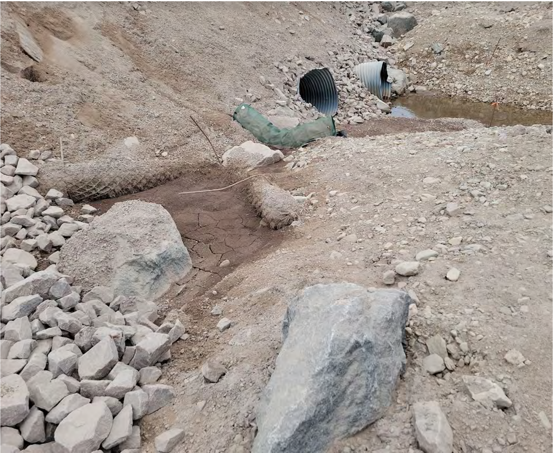
Photo 14: View of installed coconut coir log that needs the sediment accumulated upstream of it removed so that it can continue to function. As seen in the picture, it is evident that the sediment accumulation has resulted in the creation of a ramp that would make it easy for sediment laden waters to overtop the log during future sediment transport events.
