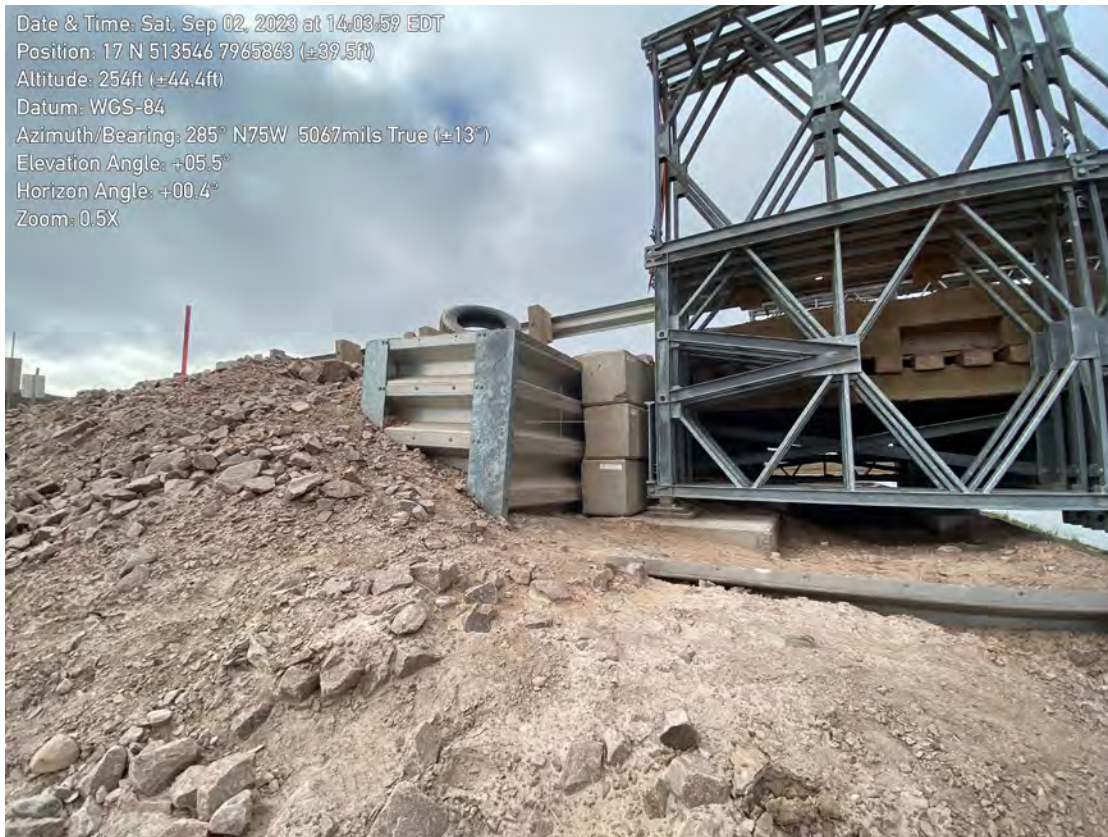
Figure 3.10: Settlement in Bridge Abutment retaining wall
