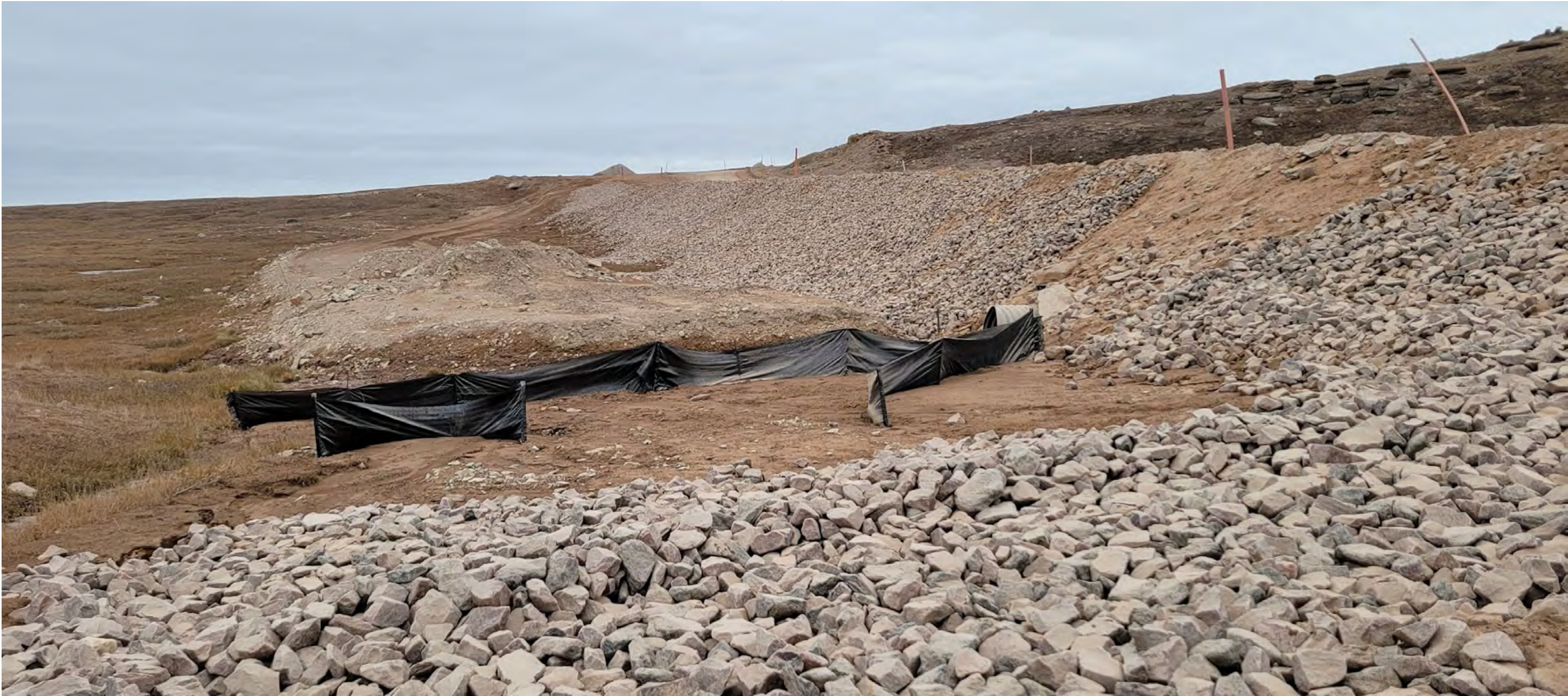
Photo 13A: Example of enhance armoring at KM74. Note accumulation of sediment on the surface or riprap above the culvert. Annual maintenance should ensure that all armoring is left in a condition that allows effective sediment management during the annual freshet,
