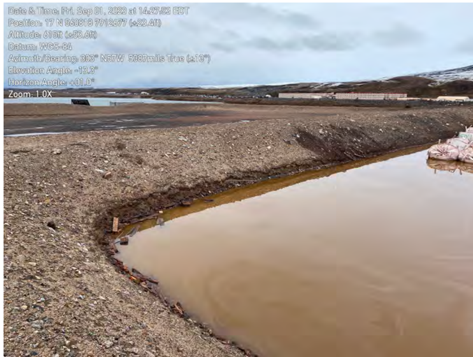
Figure 3.6: Slumping beginning on inner berm of Landfarm.
