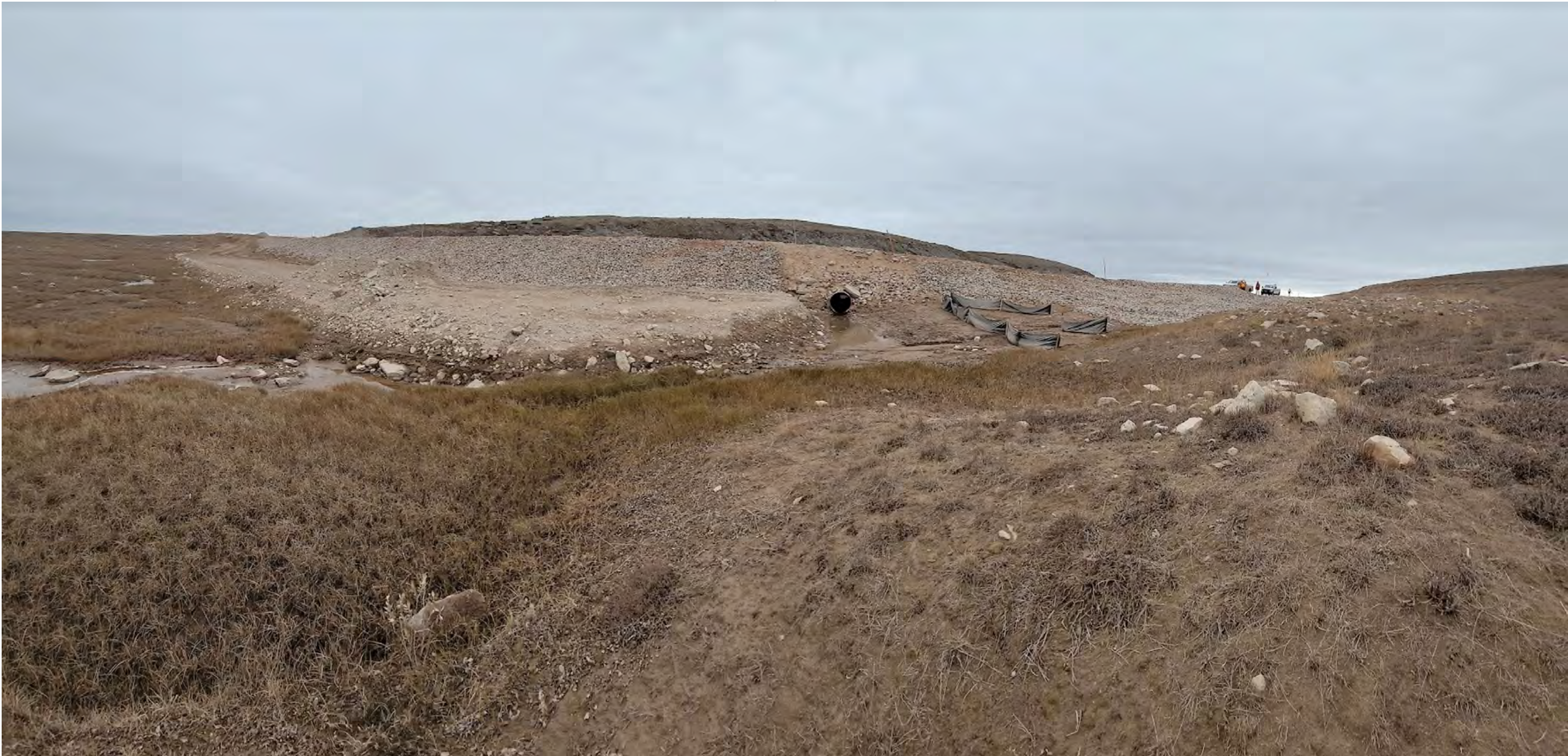
Photo 13B: View looking upstream towards culvert pictured in Photo 13A. Note that armoring appears to be incomplete with areas of exposed bare soil downstream of the silt fencing on the right side of the photo.
