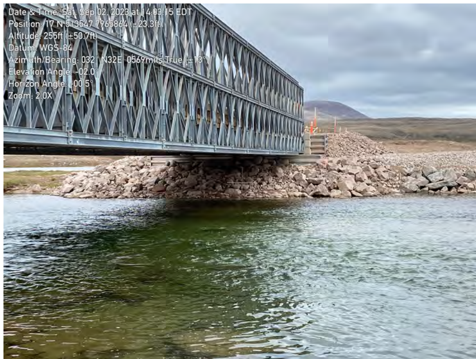
Figure 3.9: Tote Road Bridge Abutment Armouring at most northern bridge
