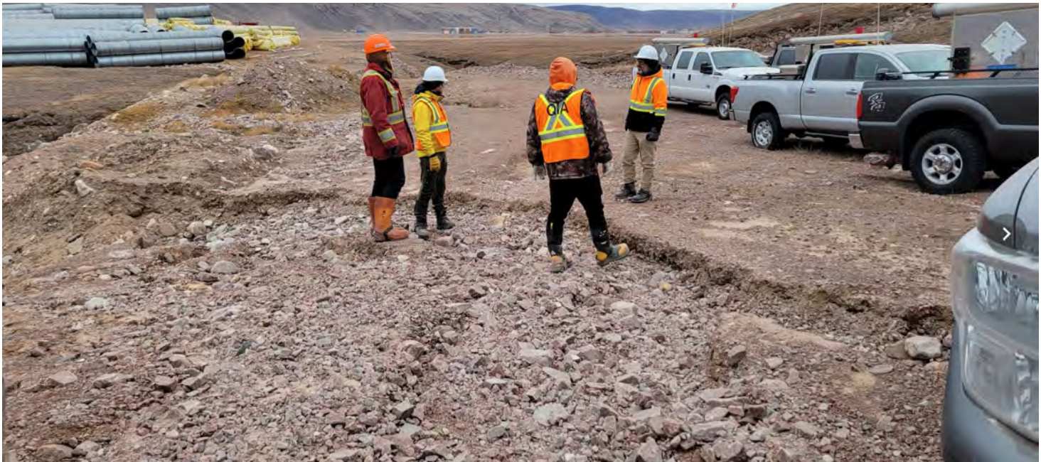
Photo 15C: View of erosion channel that has developed beneath parked vehicles at KM 7 staging area.
