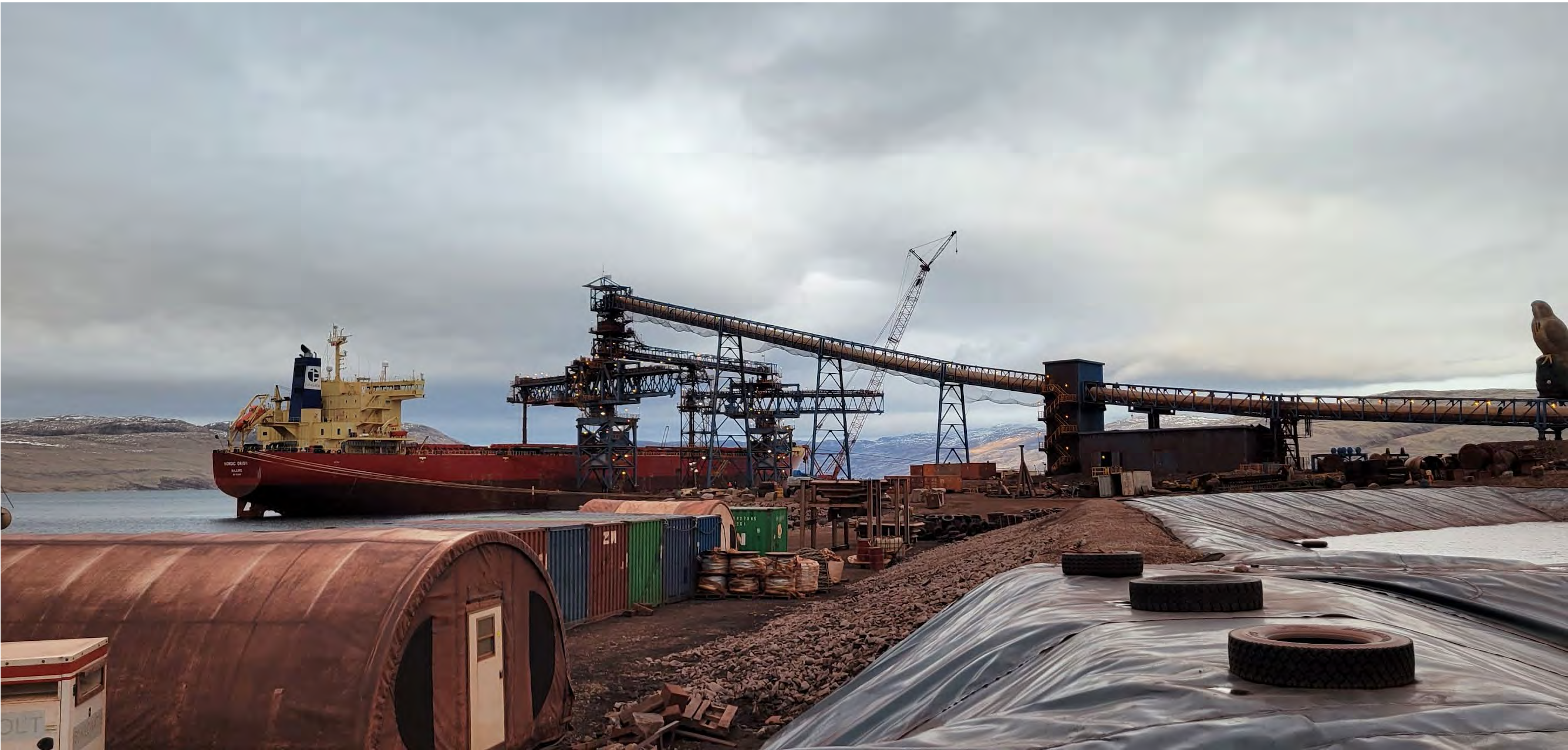
Photo 16: View (looking east) of west side of weather haven and ship loader caked with fine ore dust that has been transported by the wind from the fine ore stock pile locate south and west of the ship loader.
