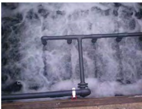
Proper air scouring in membrane tank
