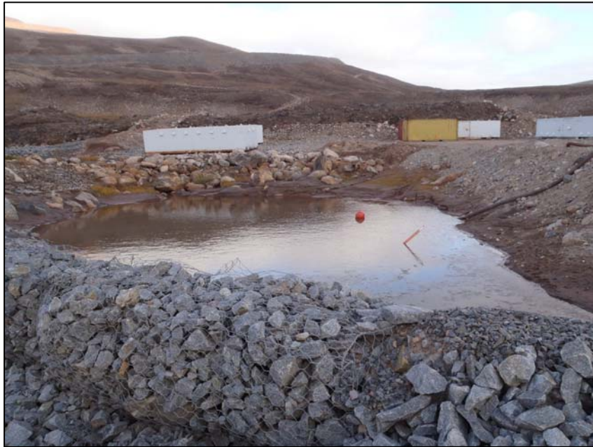
PHOTO 9 - Check dam in explosive magazine area.
