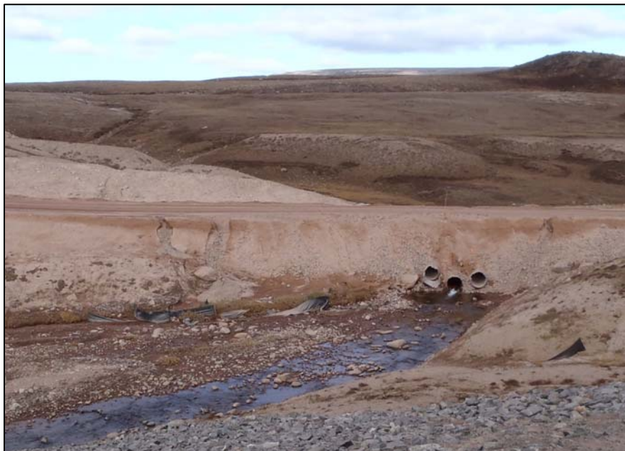
PHOTO 16 - Erosion along Mine Site Road at Tributary 3 to Camp Lake.
