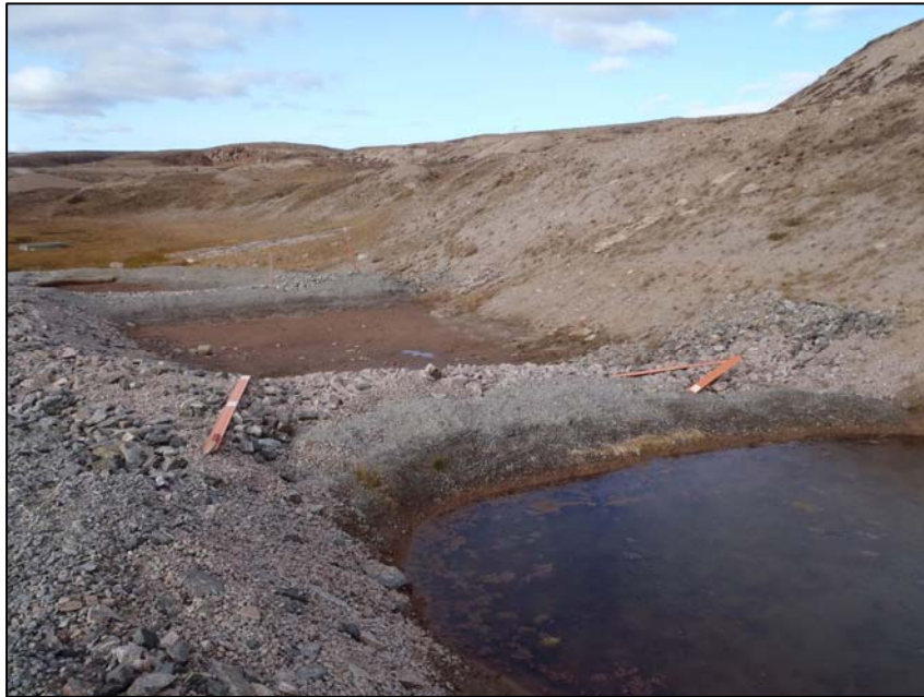
PHOTO 19 - Check dams and sediment traps by Water Jetty.
