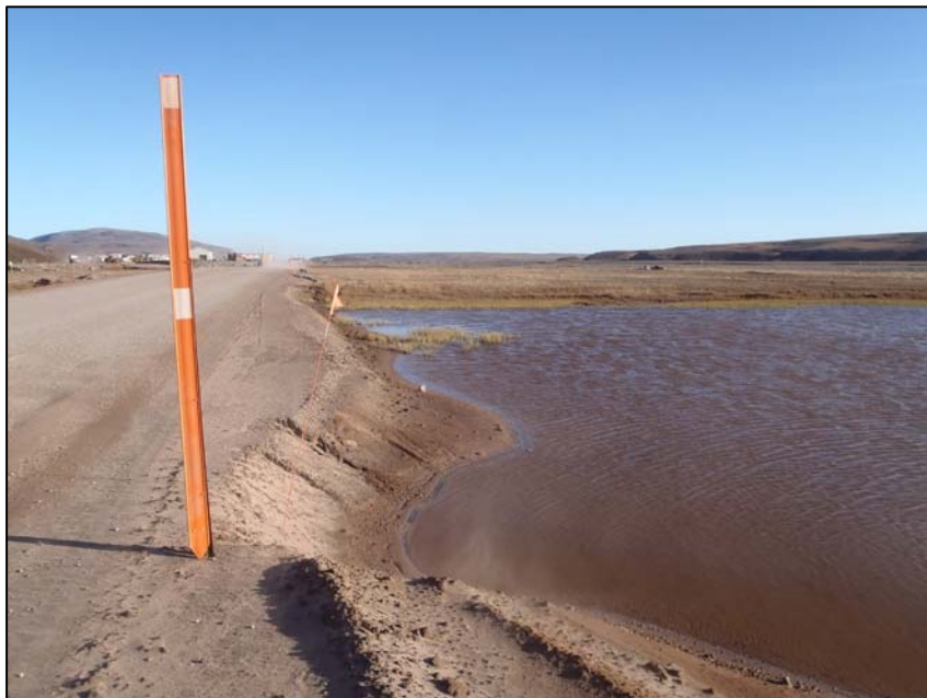
PHOTO 14 - Finer material on bank of the Mine Site Road in culvert area.
