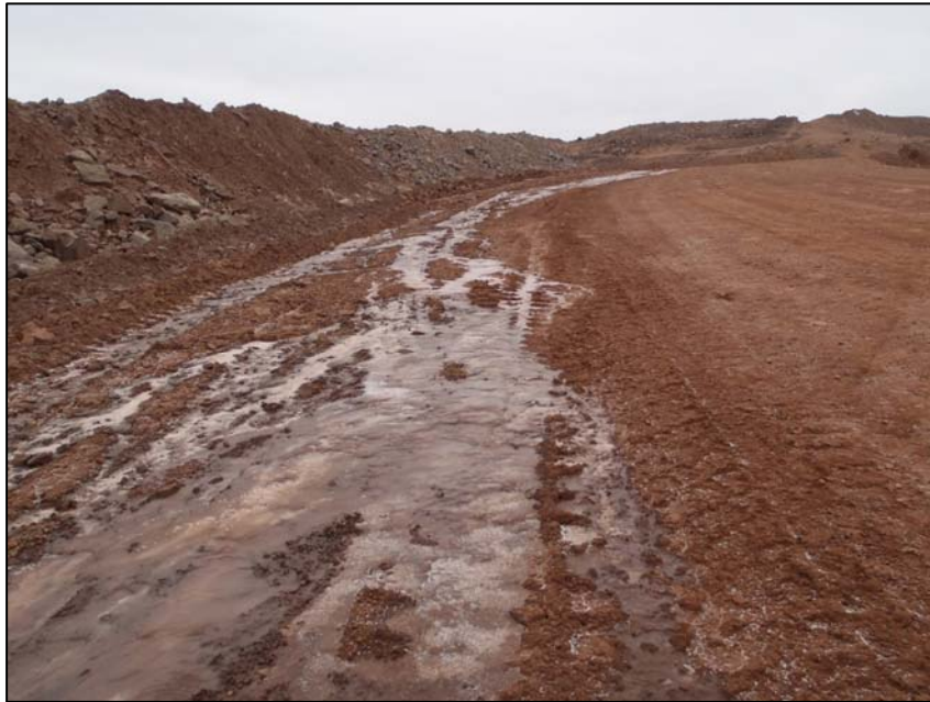
PHOTO 3 - Seepage daylighting along MHR.
