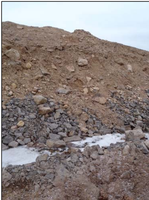
PHOTO 2 - Erosion of cut overburden slope along MHR.
