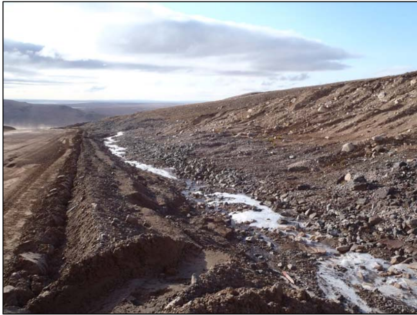
PHOTO 1 - Graded material and swale cut through material to ditch along Mine Haul Road (MHR).
