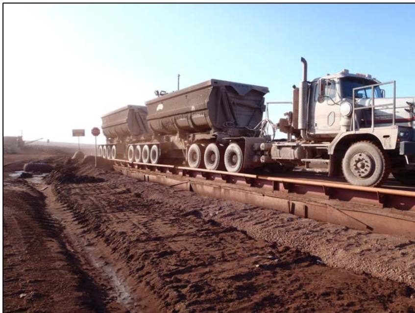
PHOTO 10 - Truck weigh scale and trench for drainage.
