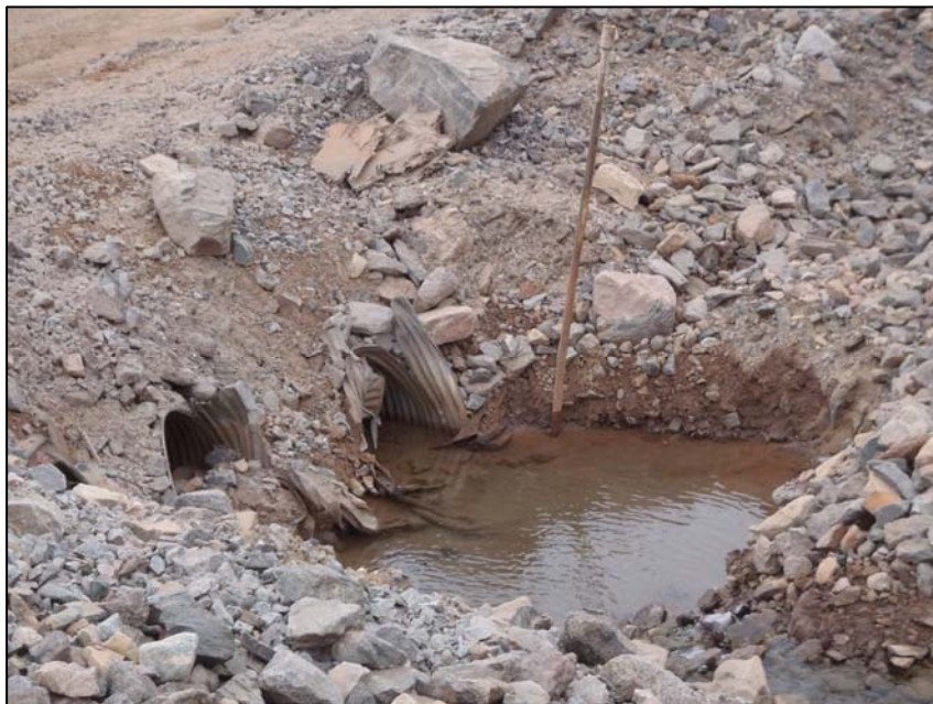
PHOTO 6 - Culvert inlet with steel rod and remnants of geotextile.
