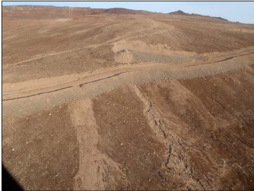
PHOTO 5 - Erosion of slope downstream of MHR culverts and cut in safety berm.
