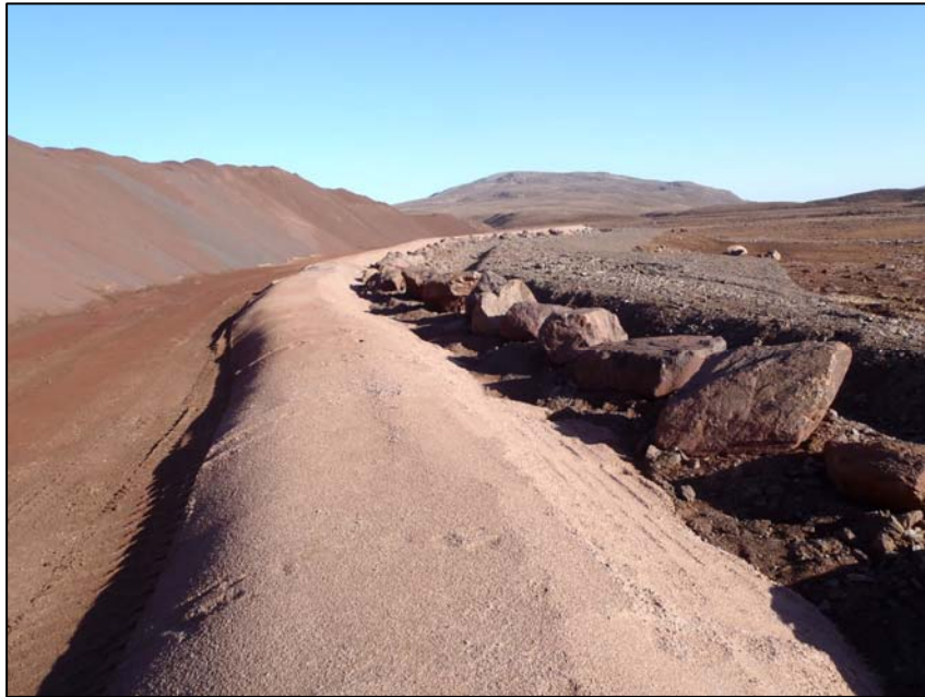
PHOTO 11 - Berm and perimeter ditch around Crusher Facility.
