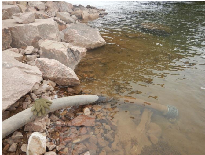
Figure 5.2 Example Water Intake at Site CV-128
