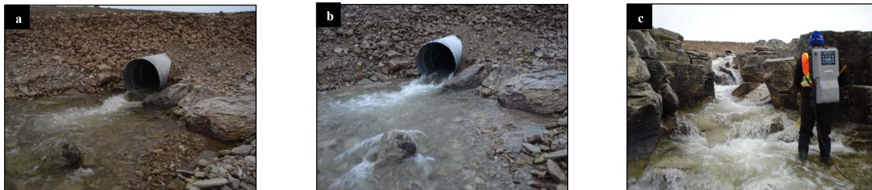
Figure 3. View from the downstream end of the culvert at crossing CV-094 during spring (a) and summer (b) 2008. View of the natural fish barrier 30 m downstream from the crossing at CV-094 (c).
