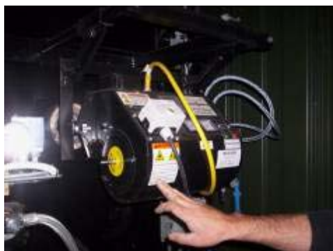
Slide out burner undo bolt
