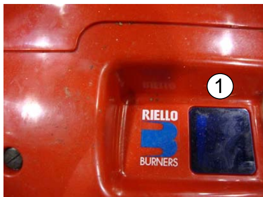
1. Primary Burner Inspection Window
