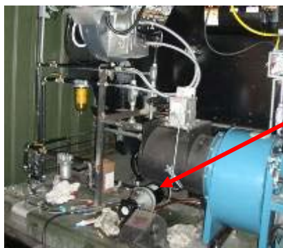
Waste Oil Burner Pump (J-Pump)
