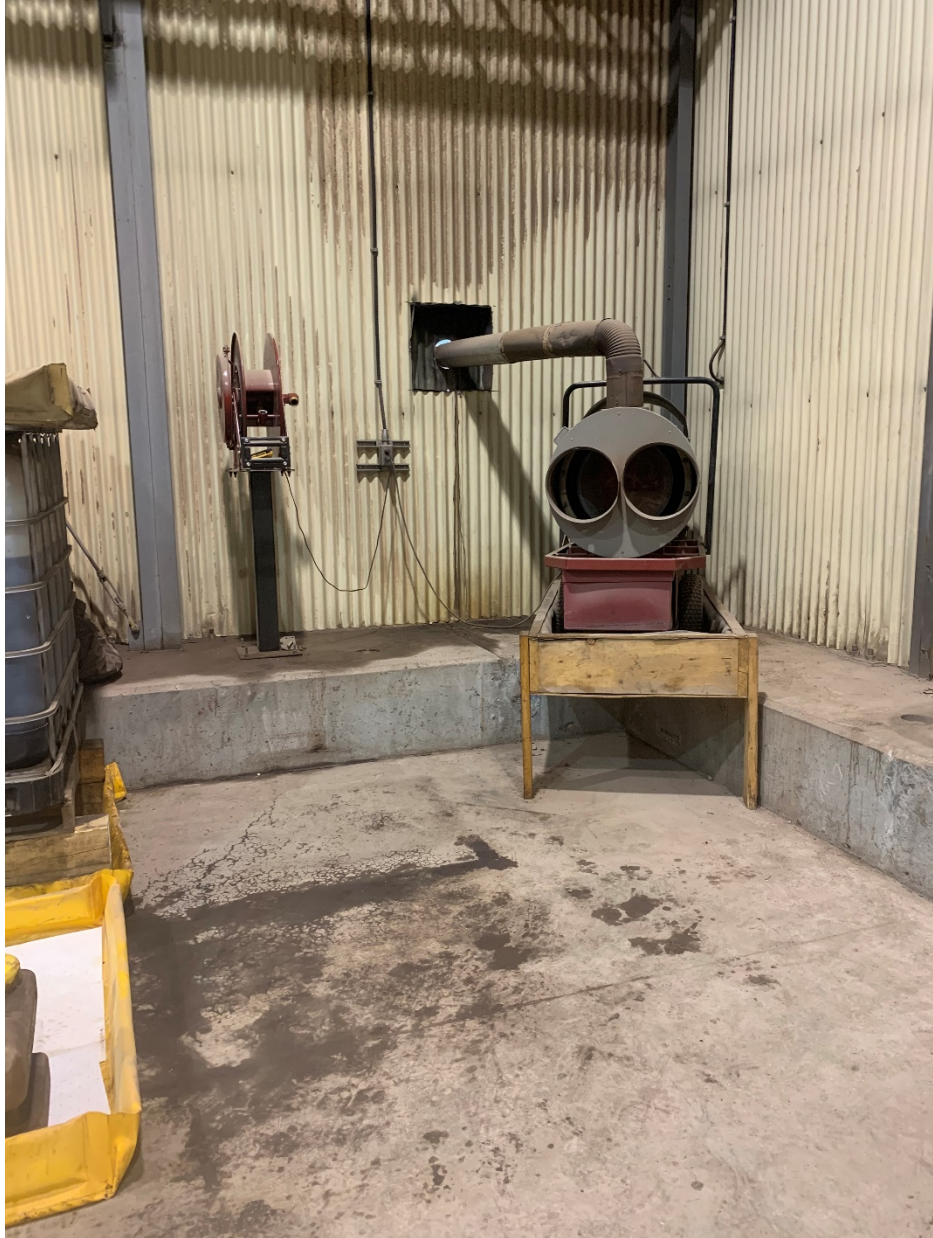
PHOTO 17 – Frost Fighter in Waste Management Building
