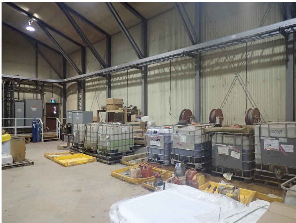
PHOTO 11 – Waste Management Building Post-August Clean Up and Installation of Tertiary Containment Under Totes
