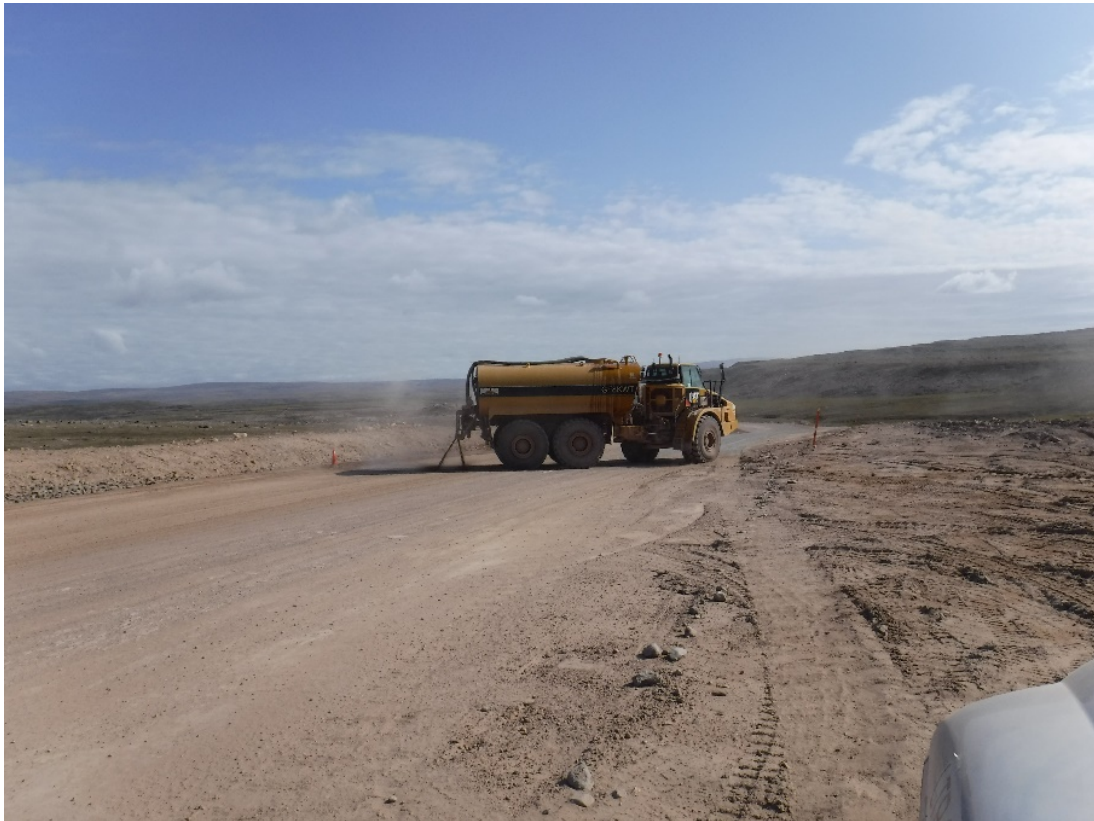
PHOTO 2 – Dust Suppression Application along Project Roads
