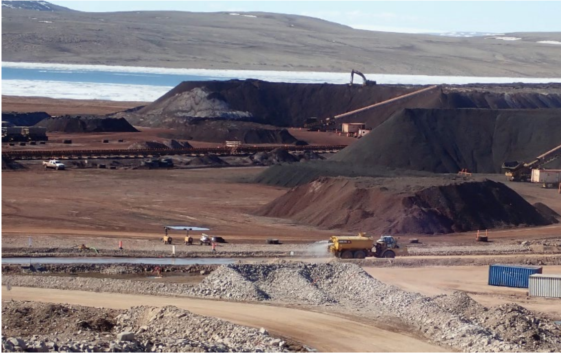
PHOTO 1 – Dust Suppression Application along Project Roads
