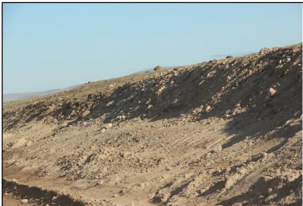
Photo 31: Erosion along the Tote Road
