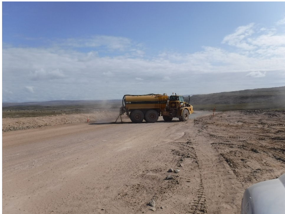
PHOTO 2 – Dust Suppression Application along Project Roads
