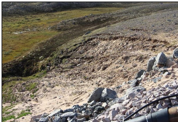
Photo 25: Unstable Terrain around the Sewage Discharge Pipe
