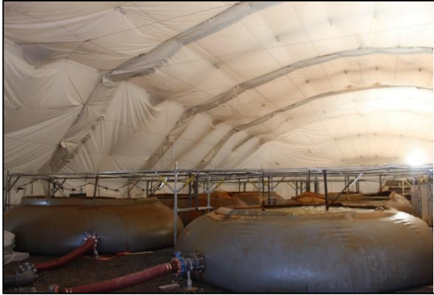
Photo 6: Chemical Treatment of Wastewater from the Waste Rock Settling Pond
