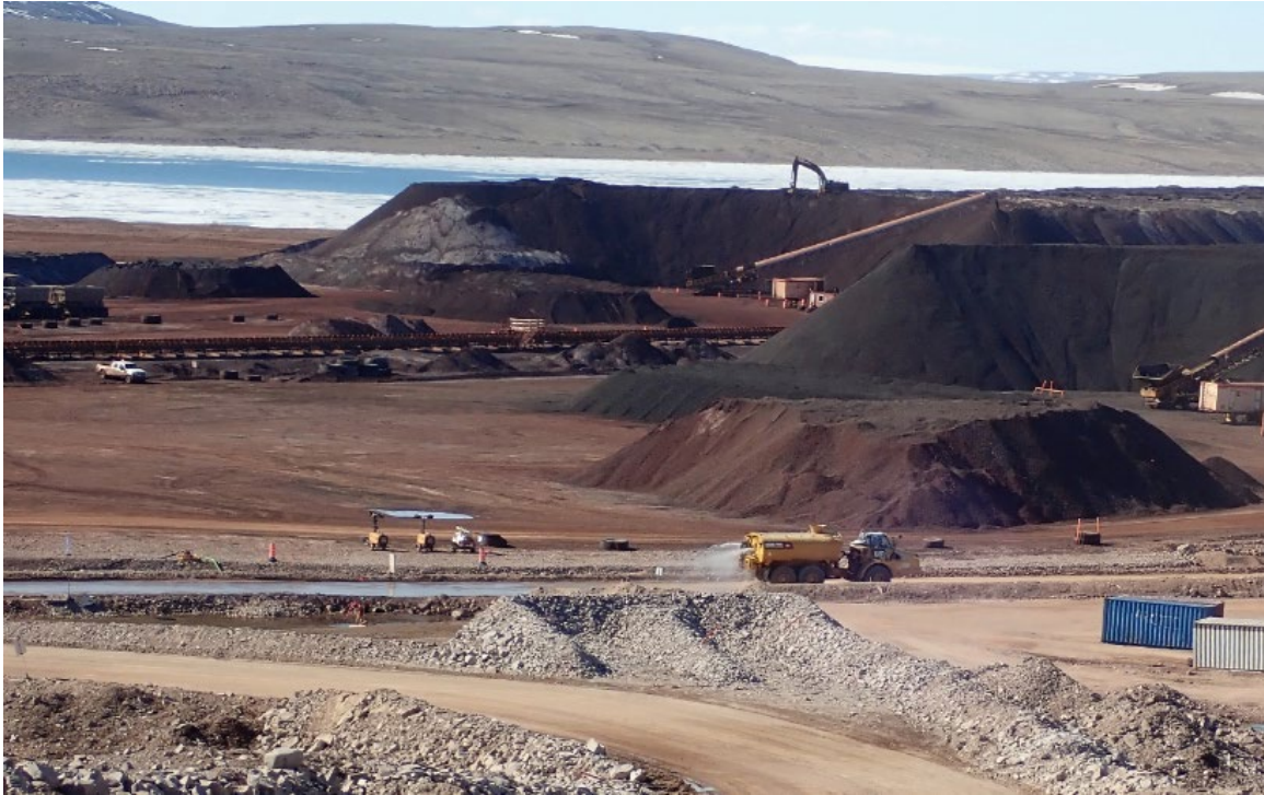
PHOTO 1 – Dust Suppression Application along Project Roads
