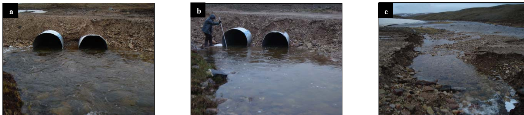
Figure 3. View from the downstream end of the culvert at crossing CV-040 during spring (a) and summer (b) 2008. View of the road washout that occurred at crossing CV-040 during spring 2008 (c).
