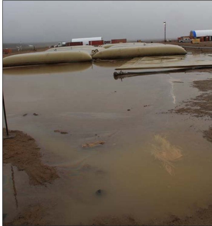
Photo 16. Pooled contact water at the fuel storage area
