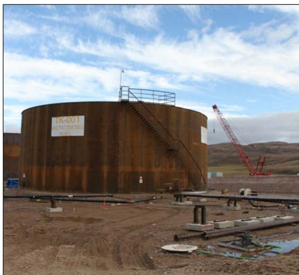
Photo 18. Pooled water in fuel storage facility
