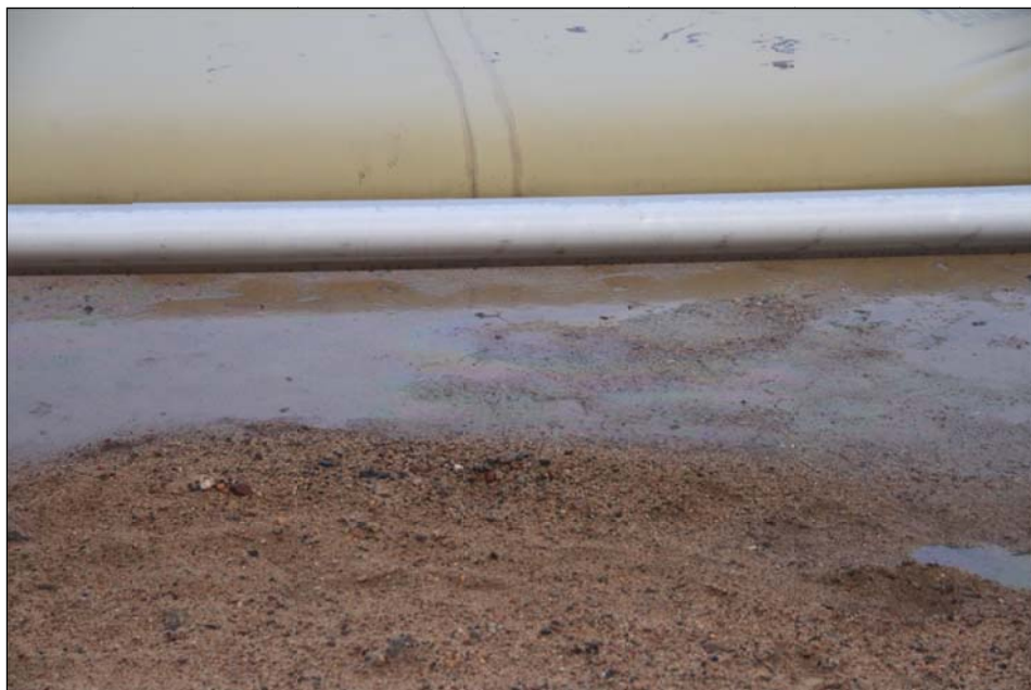
Photo 15. Evidence of fuel leakage
