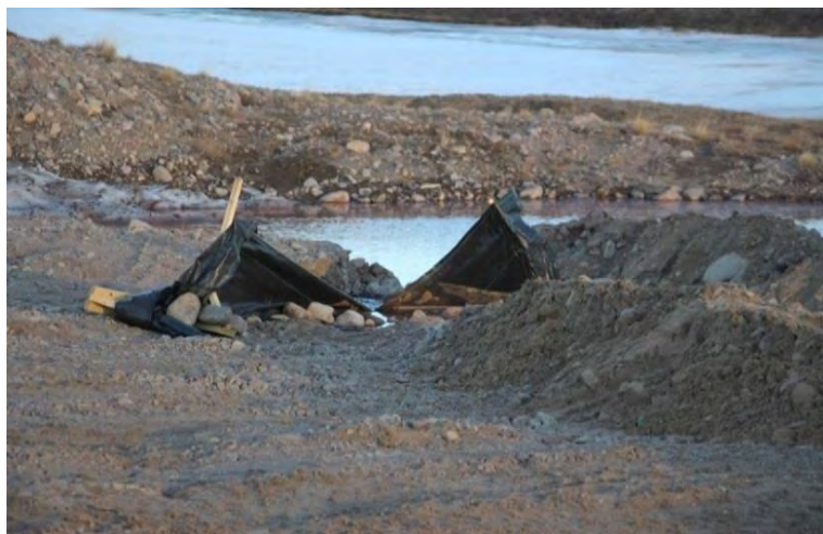
Picture 21: Deteriorated Silt Curtain
