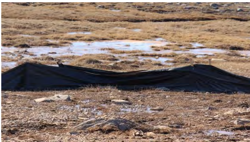
Picture 36: Degraded Silt fence
