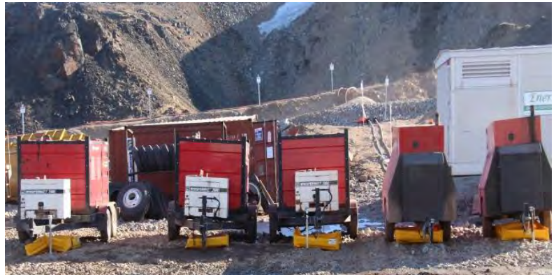
Picture 11: Generator equipped with spill trays
